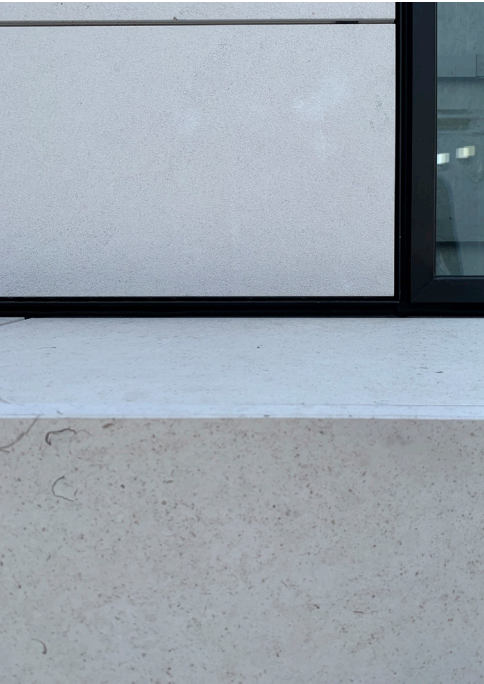
Horizontal + Vertical Grid. Moleanos Limestone. Honed Finish Thickness: 30mm Above: Hand Sample Below: Detail VMU Photograph.
