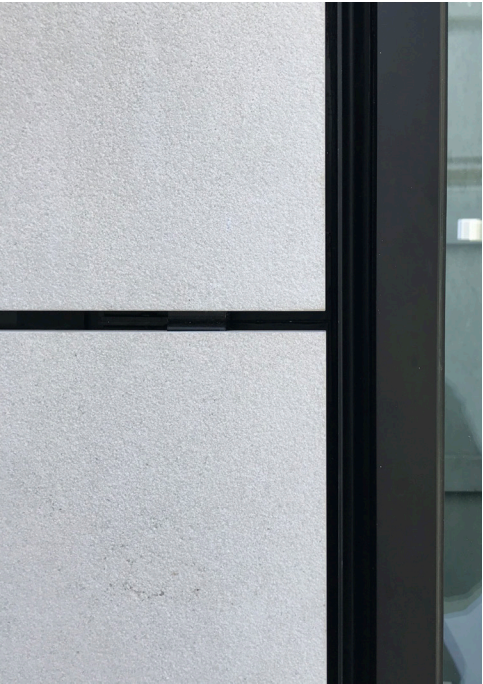
Recessed Back Panels. Moleanos Limestone. Medium Sandblasted Finish Thickness: 30mm Above: Hand Sample Below: Detail VMU Photograph.
