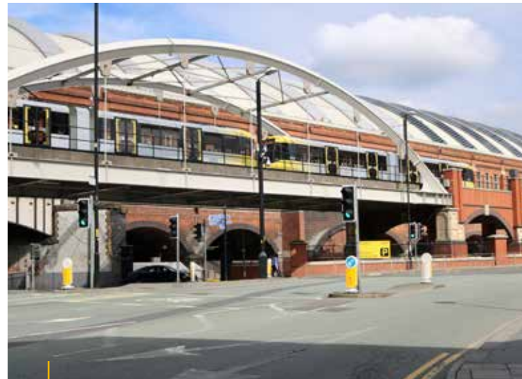
Manchester Central Roof
