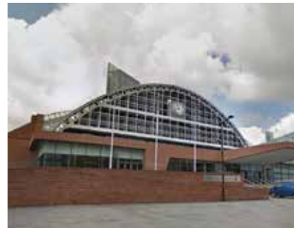
Manchester Central: A combination of old multi-brick with red sandstone base and a steel and glass vaulted structure.
