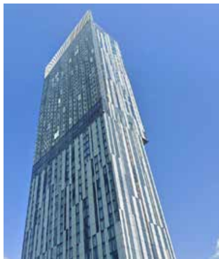
The Beetham Tower: A combination of elegantly designed glazed curtain walling, moveable glass panels and steel.
