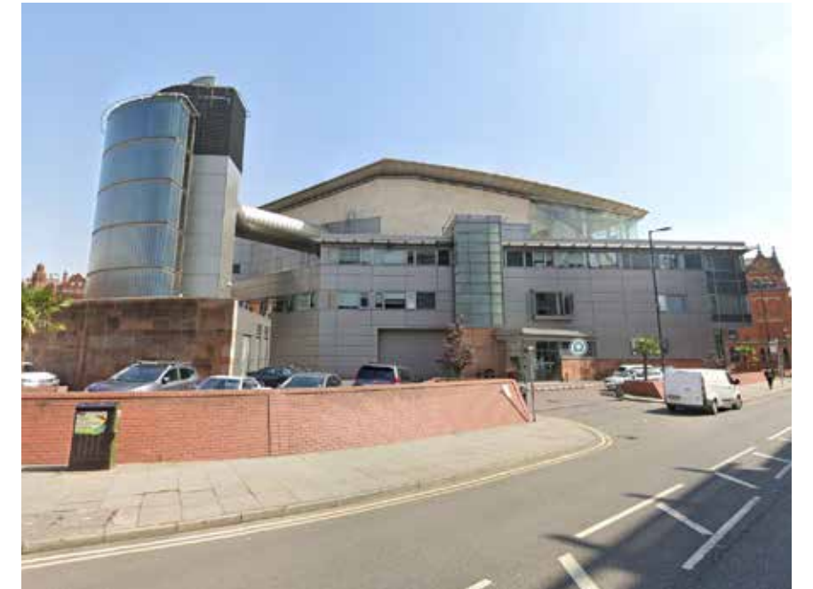
View 2 - Looking from the site towards Bridgewater Hall
