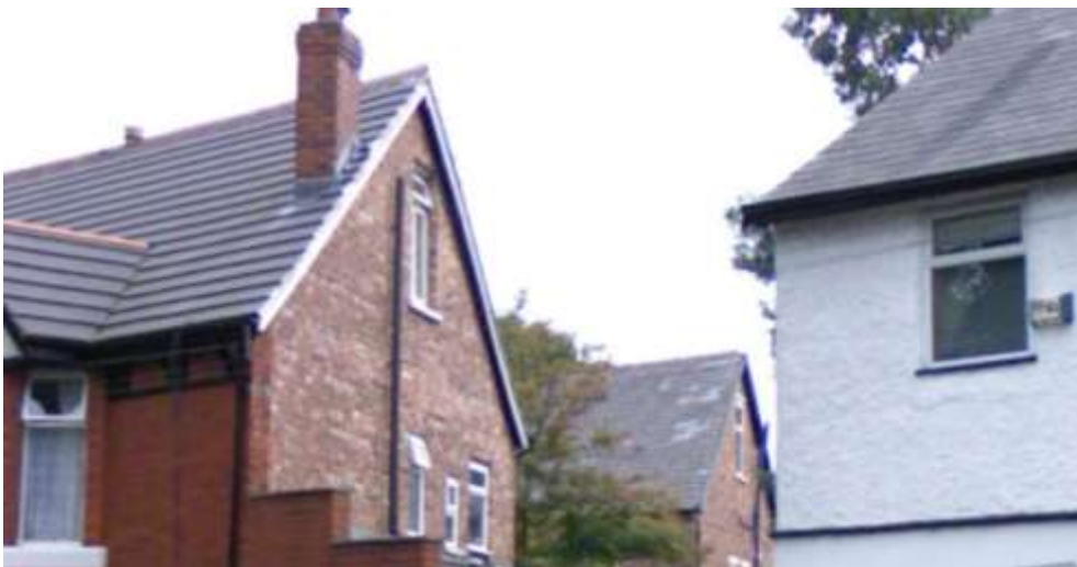
Figure 8. The windows to the side elevation of the neighbouring dwelling serve non-habitable rooms
