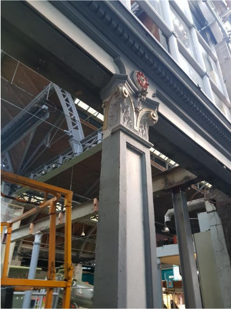
Fig.05 – Photograph of decorative cast iron beam
