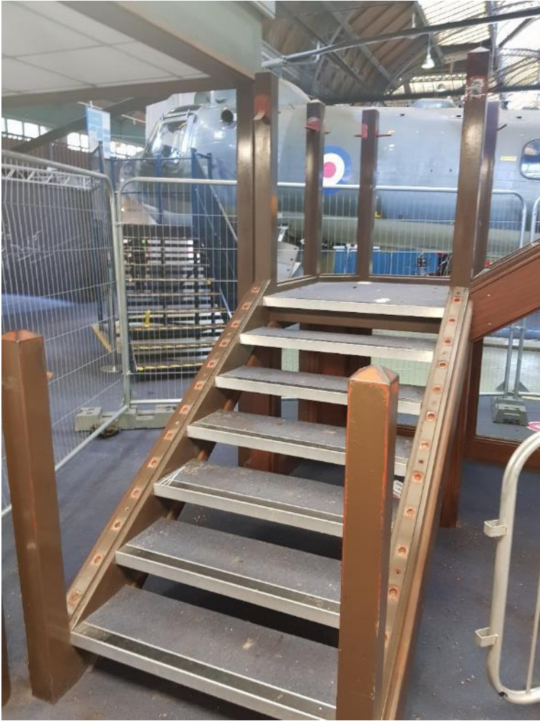
Fig.07 – Photograph of staircase components being removed
