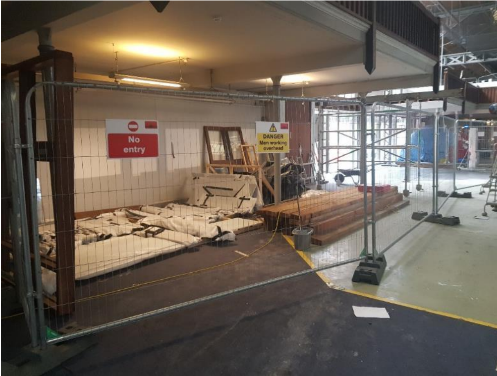
Fig.08 – Photograph of tagged, protected and stored elements and components
