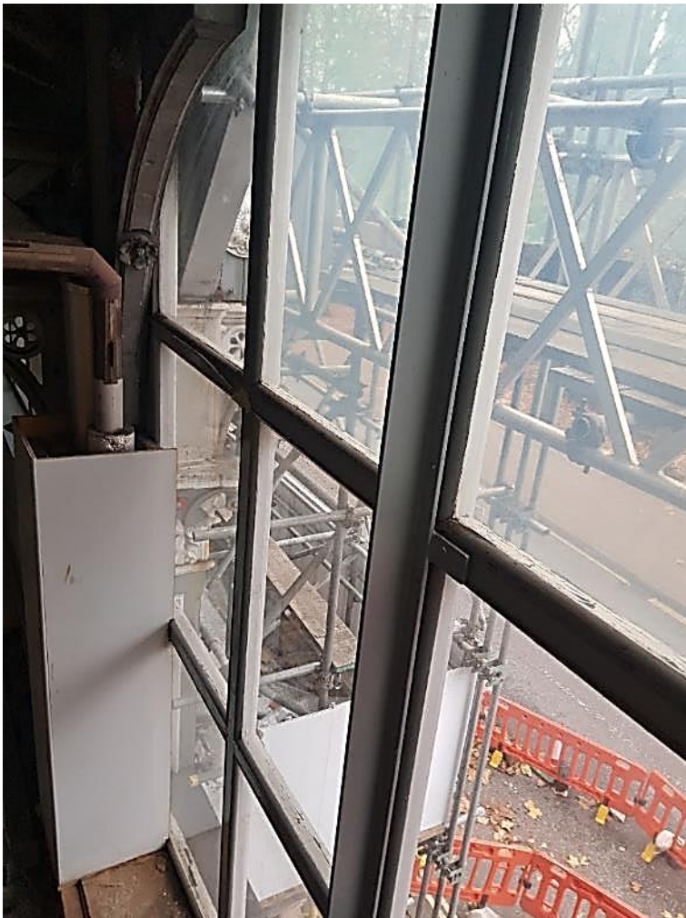
Fig.02 – Photograph at high level with 'T' section
