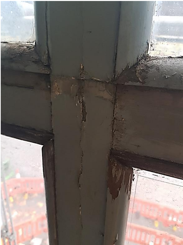
Fig.01 – Photograph at intersection of mullion and transom
