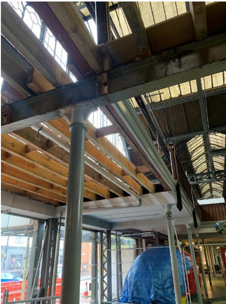
Fig.03 – Photograph to the underside of Mezzanine floor
