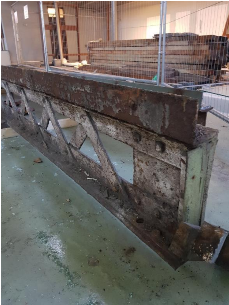
Fig.04 – Photograph of lattice beam
