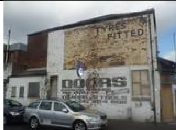
P5: Gable end of 786 Stockport Road. Spray painted business services indicating former use of the building. (Tyre Fitting/Doors)
