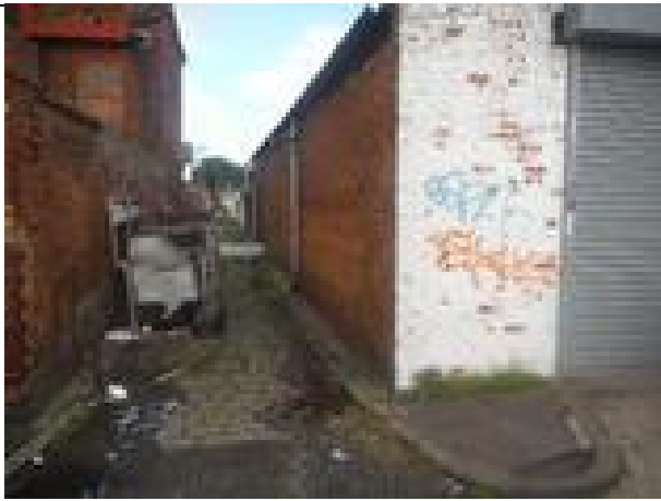
P1: A series of attached single storey units occupy the west of the site (rear of the residential properties)at the site
