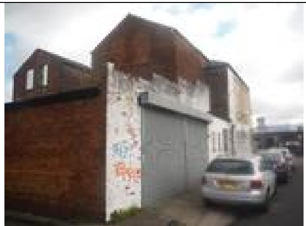
P2: Single Storey unit to rear of 786 Stockport Road.
