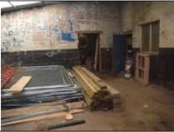
P8: Stored construction materials were present within the interior of the properties
