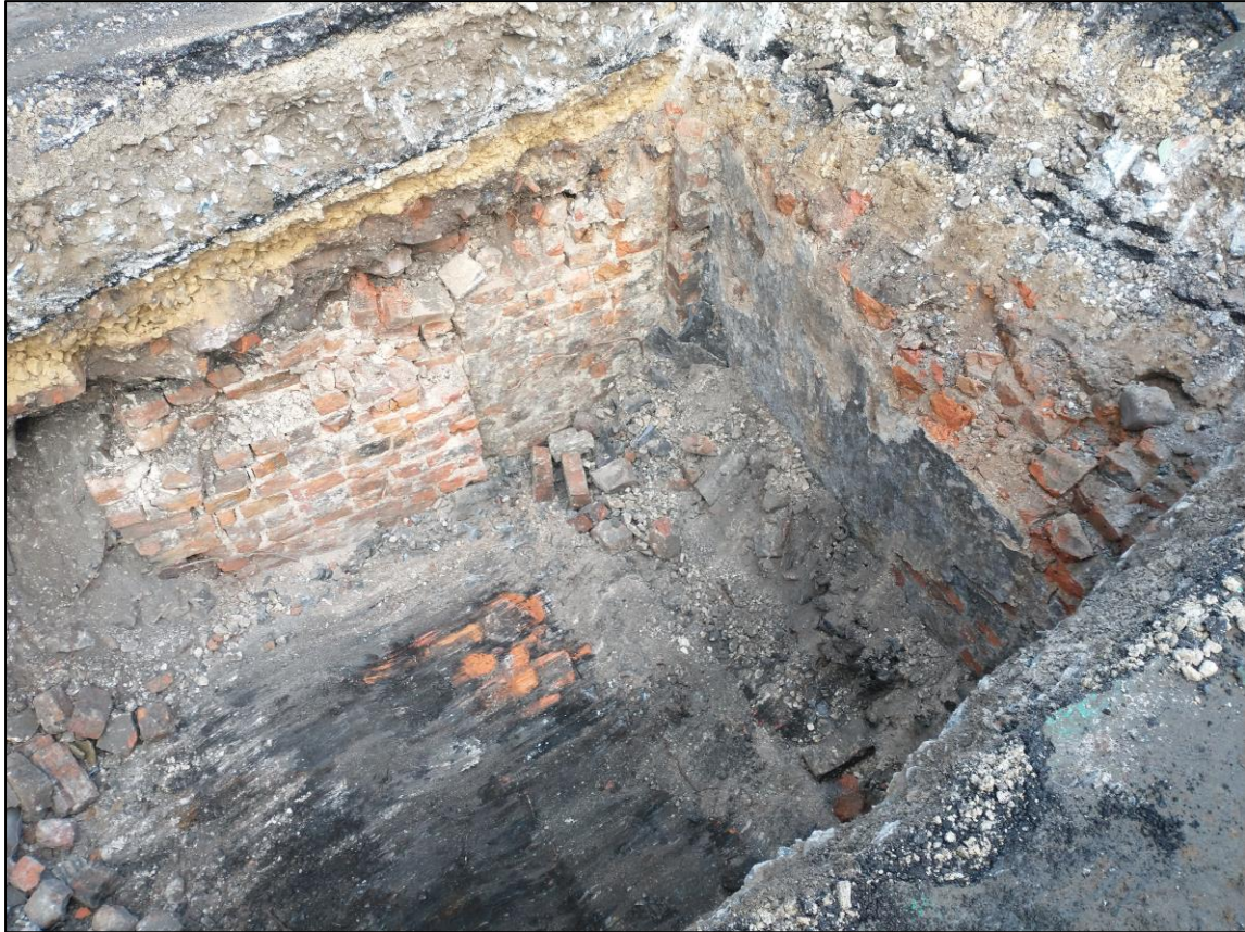
Plate 10: Wall 308 and floor 309, note blocked doorway at top centre of photo, looking southwest
