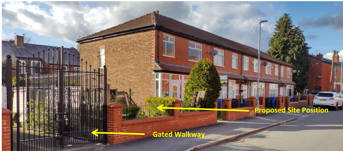
Street view showing site position, existing adjacent property, neighborhood and context.
