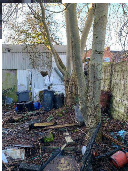
Fig.15: Front and interior of the yard area at the north end of B2
