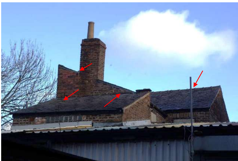
Fig.7: B2 West elevation, showing complex roof configuration, arrow shows examples of potential; roosting features.
