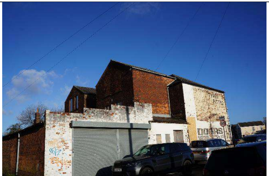
Fig.2: South elevation of the site, showing the single storey lean-to extension that runs along the rear of the buildings and two full height extensions at right angles to the main building.
