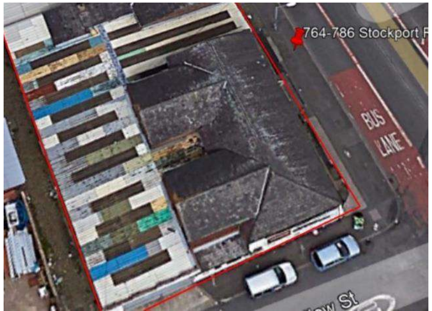
Fig.3: Google Earth Pro image of roof configuration B1
