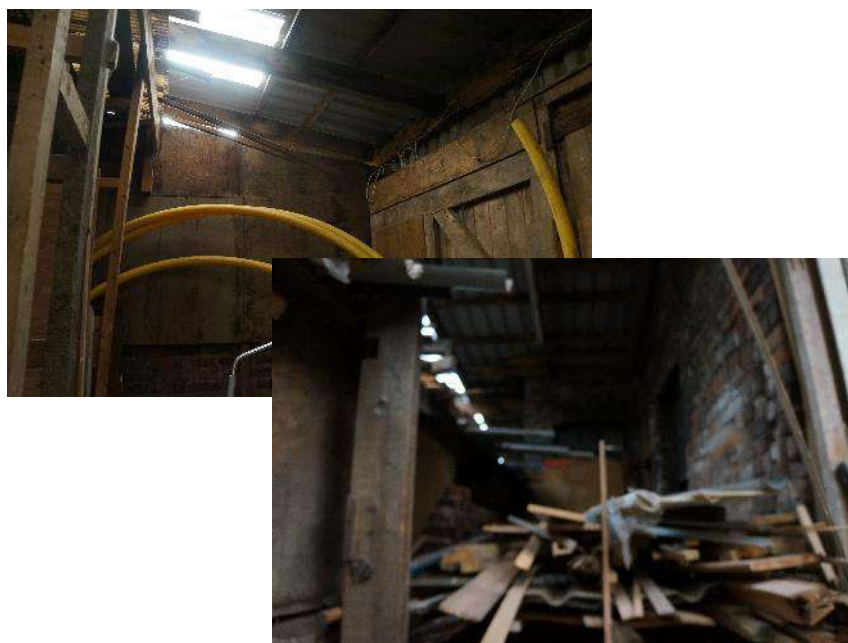
Fig.13: Interior of the single storey lean-to area.
