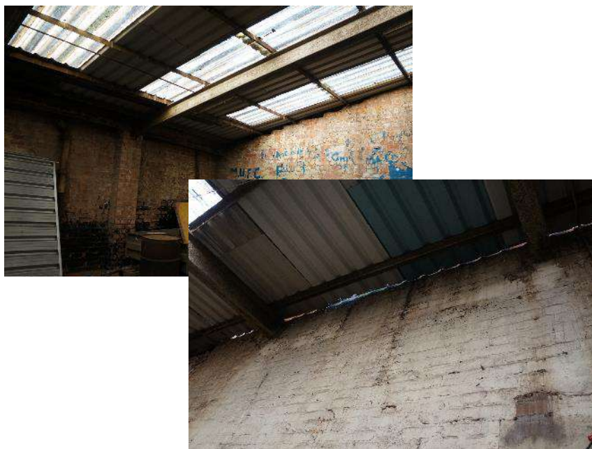
Fig.12: Interior of the single storey lean-to area.
