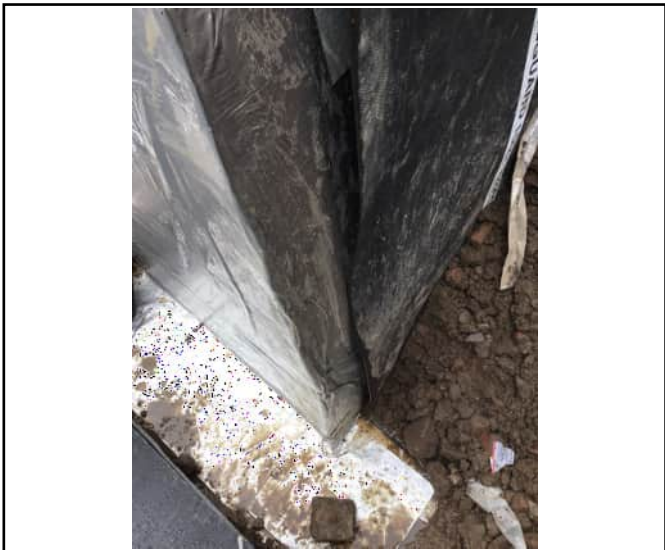
Final corner of D5 complete
