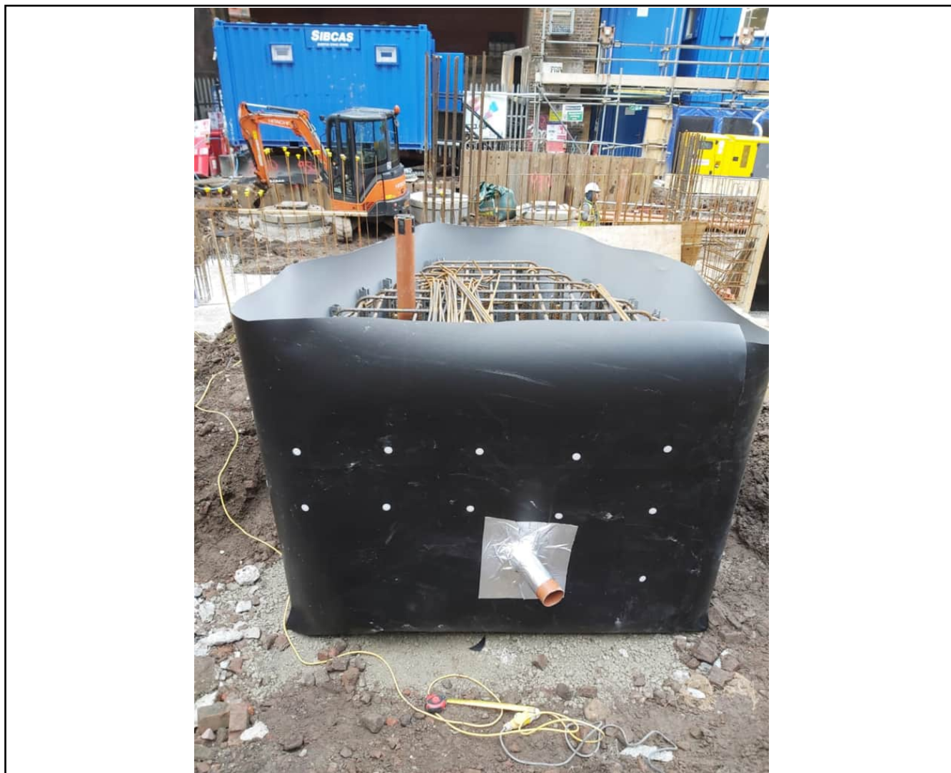
Overview of pile cap sealed
