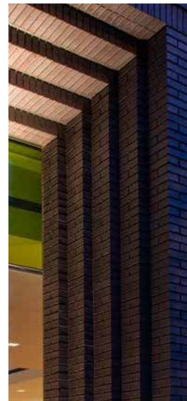
F Bond: Stretcher (corbel detail)
