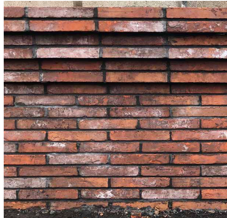
1 Stack bond corbel detail
