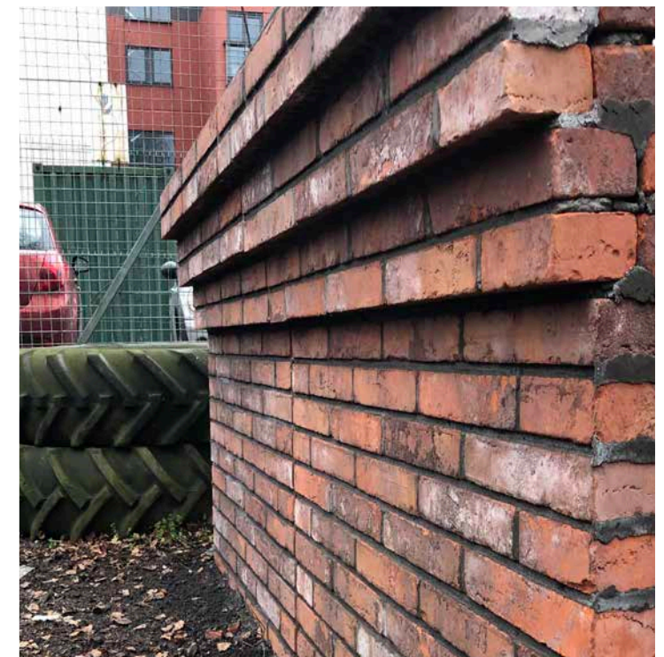
2 Stretcher bond corbel detail
