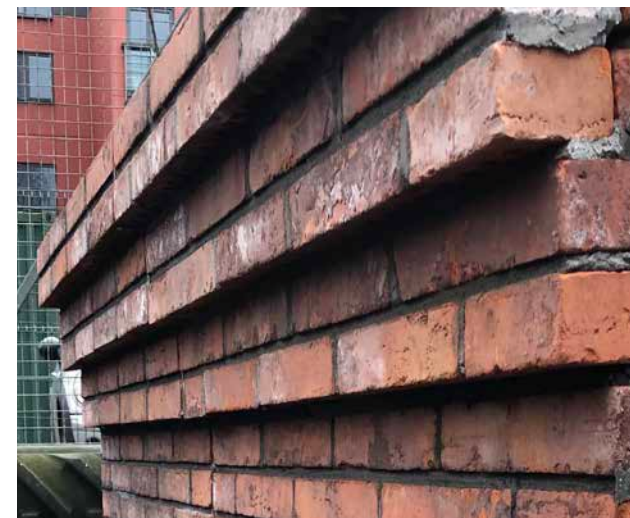
F Bond: Stretcher (corbel detail)
