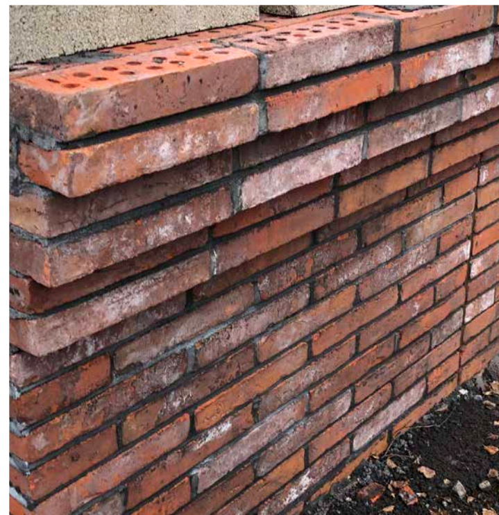
1 Stack bond corbel detail
