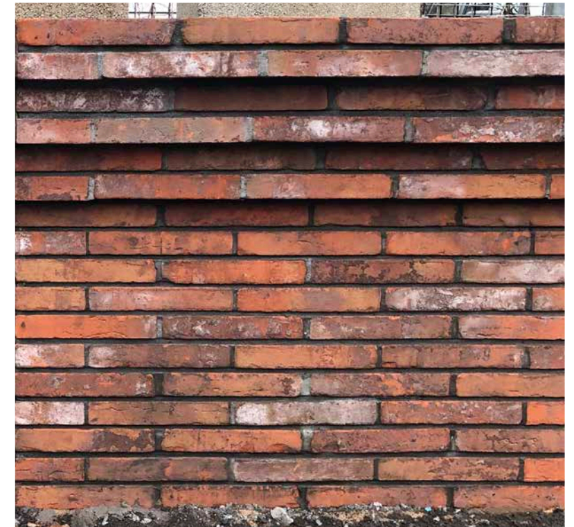
2 Stretcher bond corbel detail
