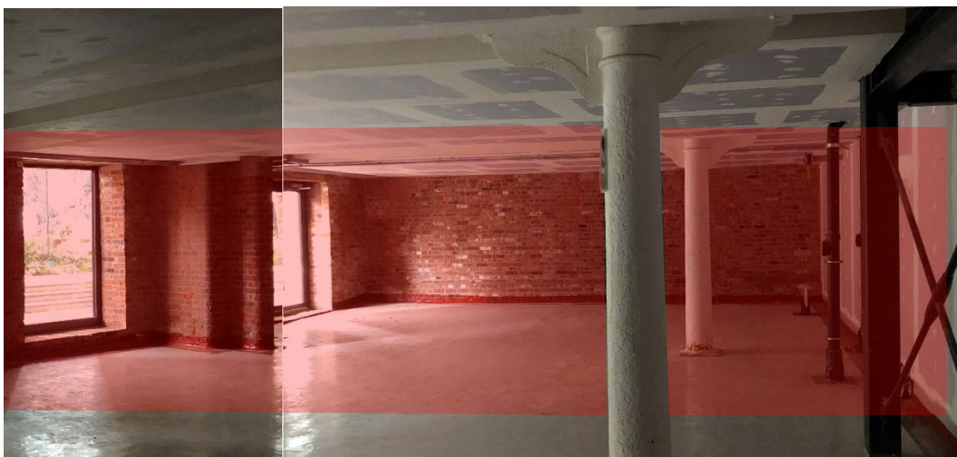
Figure 8: A view looking south-east into the unit (background) from the adjacent unit in the foreground. The red shaded area denotes the approximate location of the party wall between the two units.
