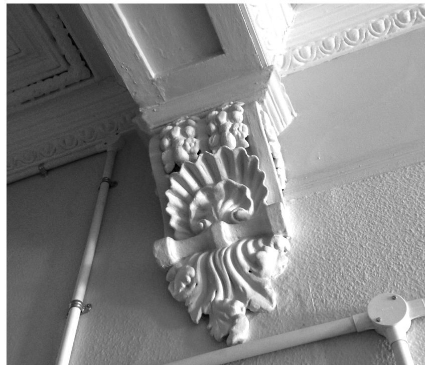
Hallway ceiling 2014 condition
