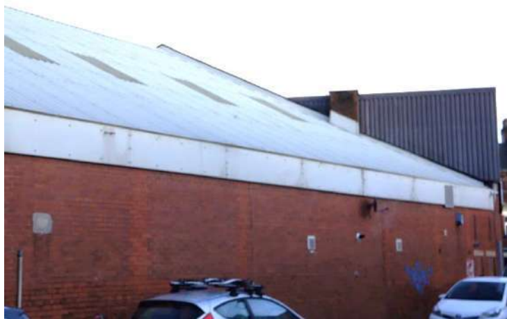
Fig.2: South elevation of the site, showing the corrugated sheet roof and cladding to the fascia of the frontage.
