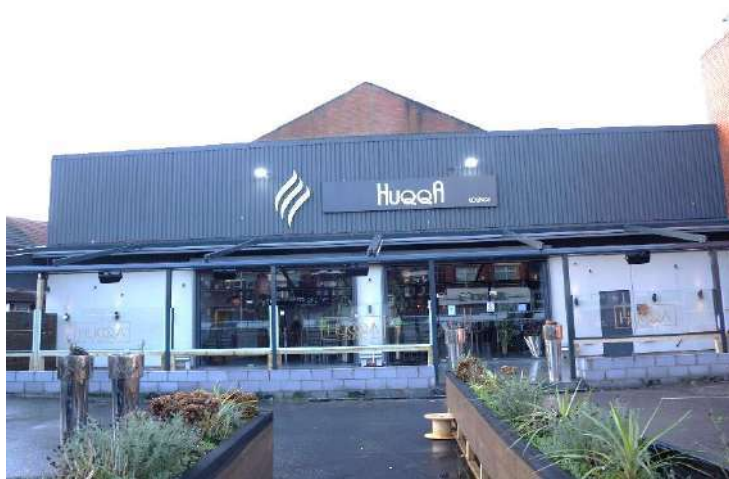
Fig.1: Eastern (road front) elevations of the restaurant
