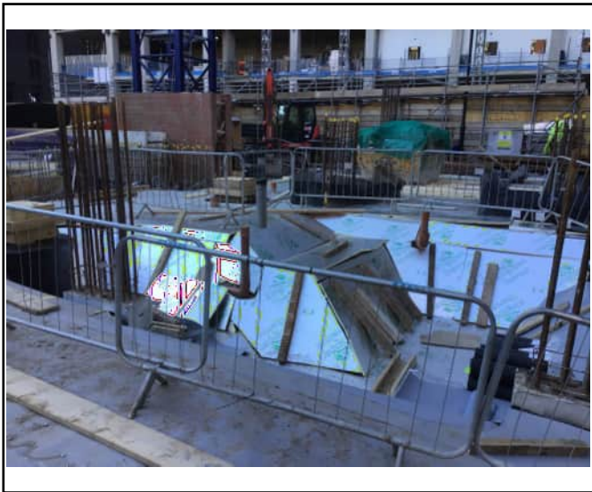
Overview of Gridline 5-7 being
