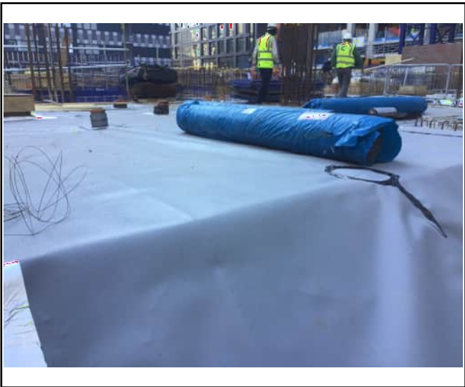
Overview of verified section
