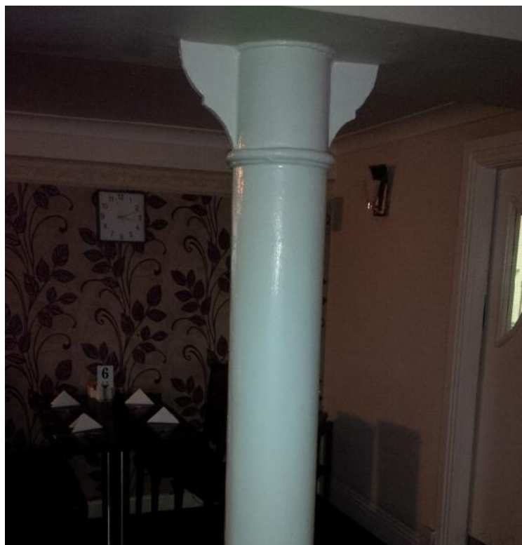
Figure 9) Cast iron column
