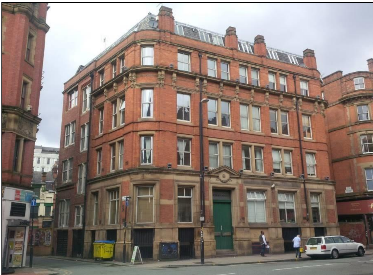
Figure 5) Kingsley House facade (13/15 Newton Street)
