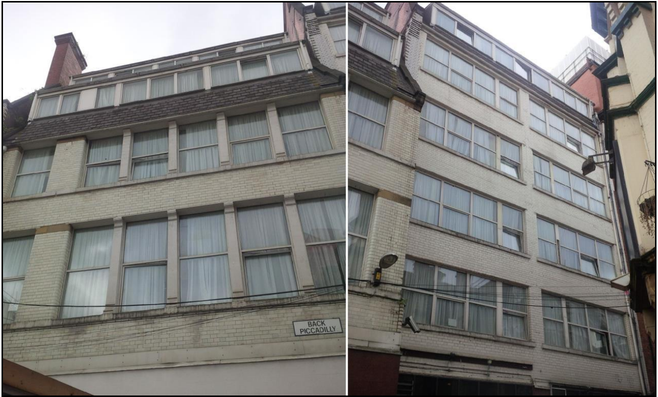
Figure 7) Back Piccadilly facades of nos 55/57 and nos 51/53
