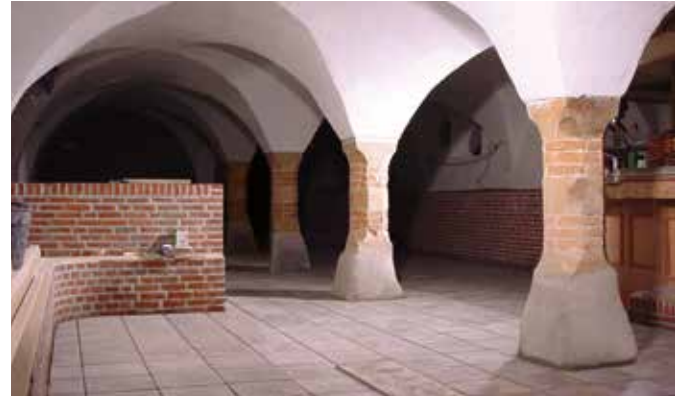
Typical damage through salt efflorescence.
