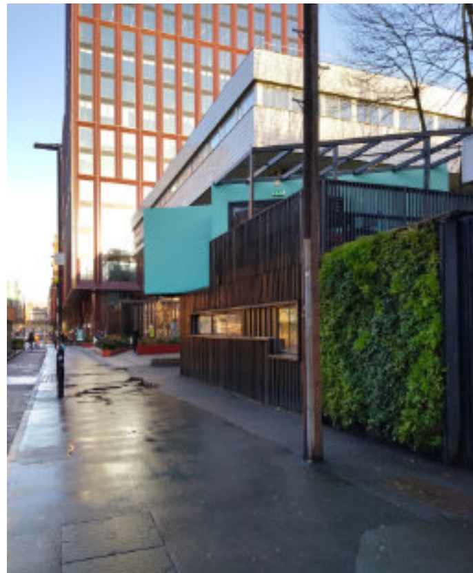
View North along Oxford Road towards Manchester Technology Centre
