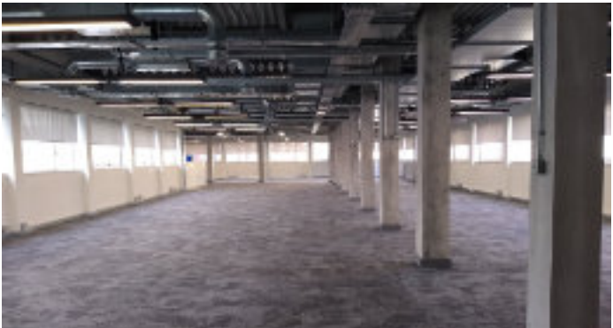
Example of Existing Third Floor Fit-Out
