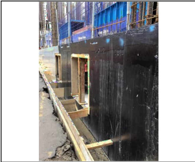
Primed concrete wall on
