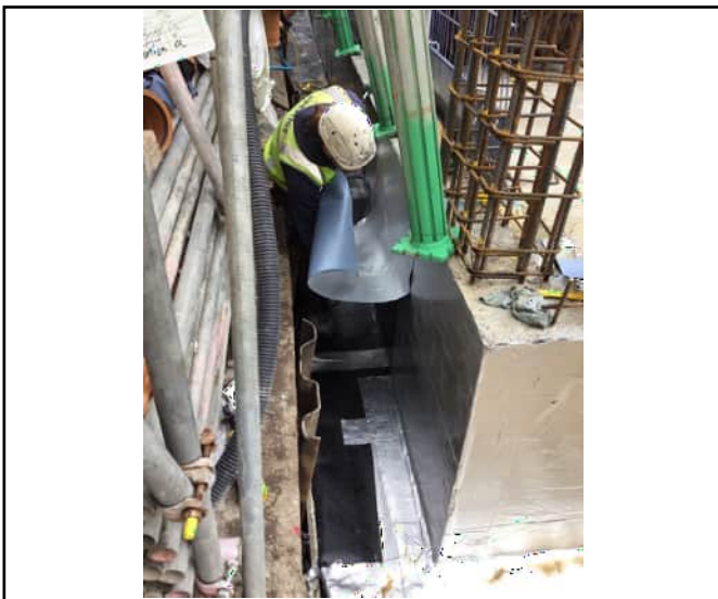
GR SAM applied to southern toe
