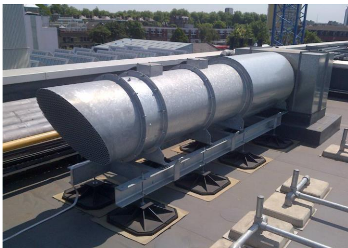
Figure 2 - Typical Smoke Fan Arrangement
