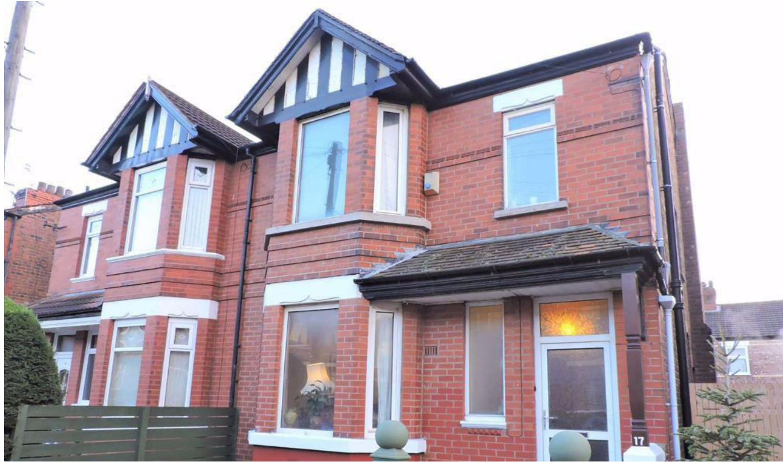
a. View of the Front facing north showing the adjacent property.
