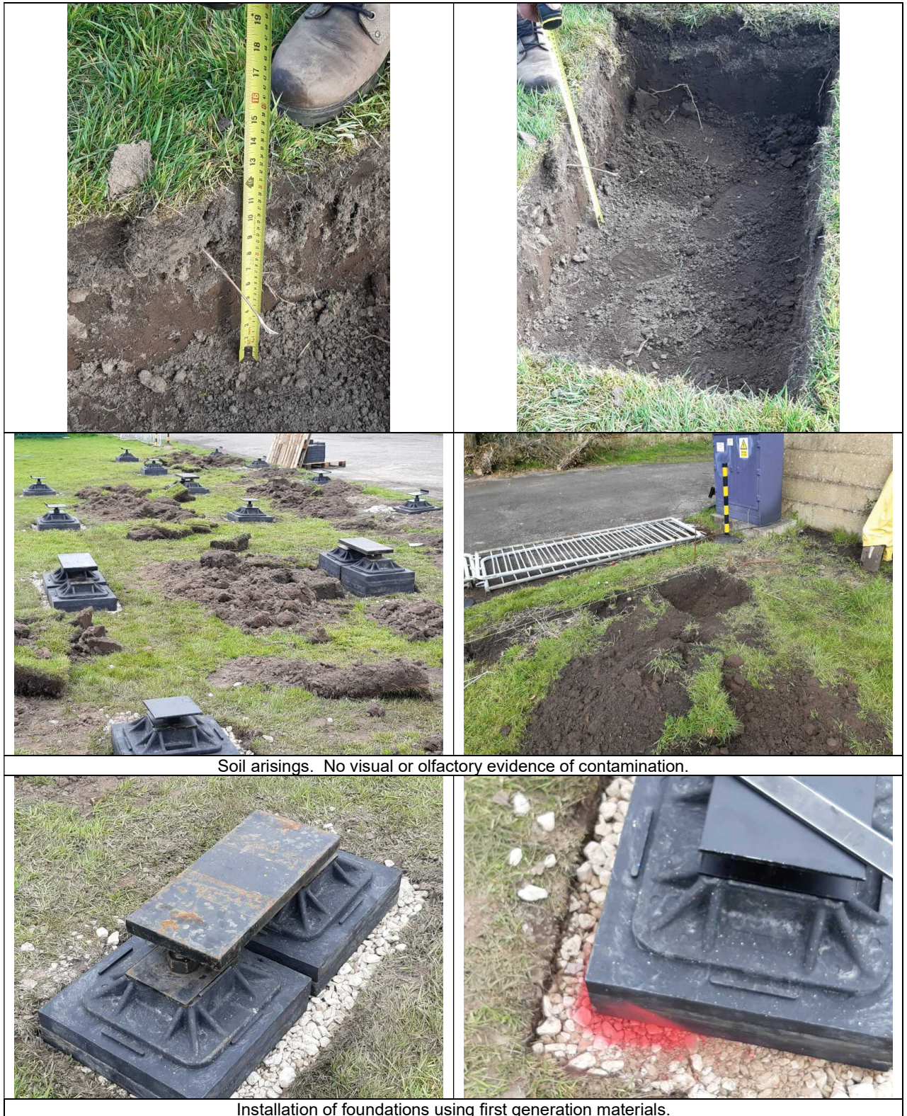
Plate 4-3: Excavations for foundation installations.
