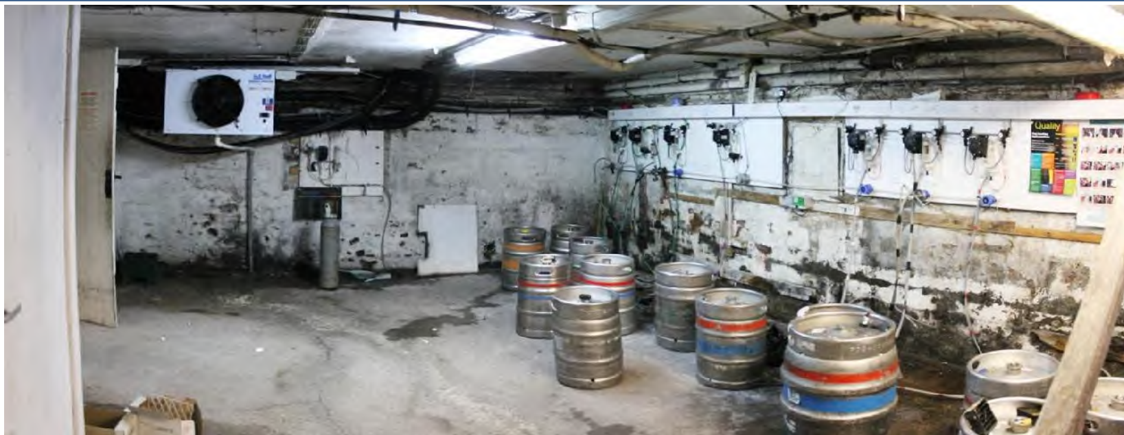
Photo 13: Main club building basement area 1
