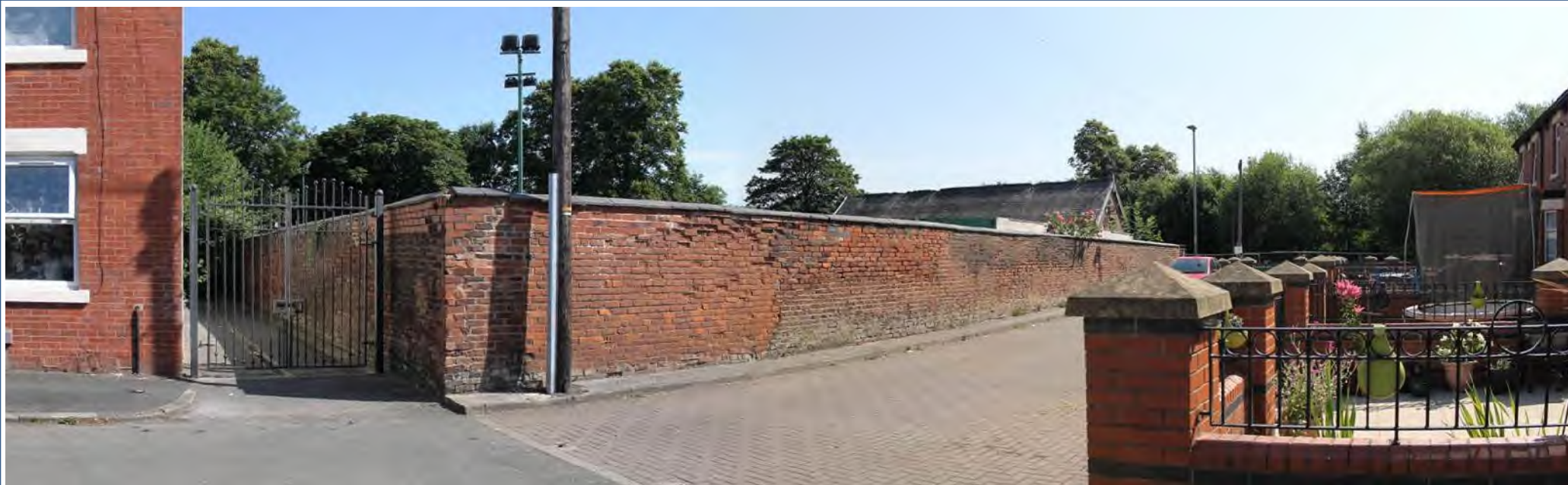
Photo 3: Site boundary wall from Backwell Street looking north
