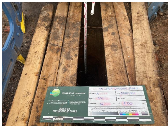
Soakaway Pit 1: Internal view of excavation
