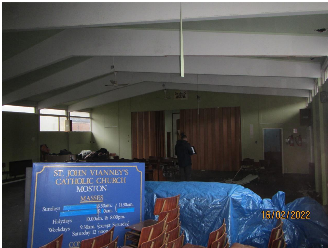
Photograph 11 – Looking south-west within the main hall of the building, showing the high levels of natural light entering through large windows and the doorways to the backrooms.
