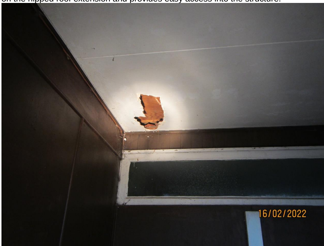
Photograph 8 – A gap located at the eaves within the building's porch, assessed as being unsuitable for bats as its positioning restricts access for bats.
