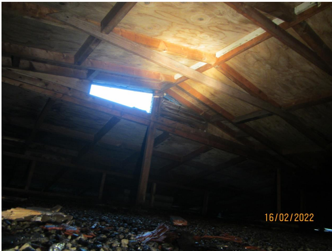
Photograph 13 – Looking north-east within the hipped extensions loft void, largely unsuitable for bats, with single skin plywood timber, rafters, and all external features visible from within and exposed to high levels of natural light.
