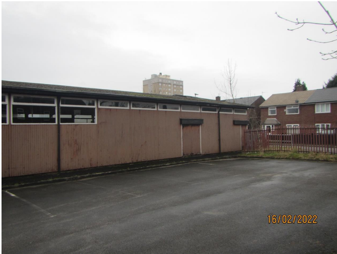
Photograph 5 – North-western aspect, showing the primary pitched roof, wooden cladding, large windows in timber frames and fire exits with timber fascia all tightly sealed.
