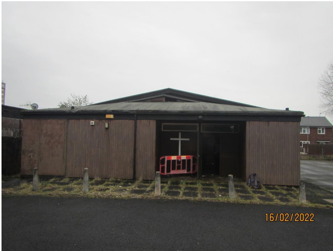
Photograph 1 – The north-eastern aspect of St. John Vianney Presbytery, with pitched roof and hipped extension clad with bitumen roof membrane and various timber features
