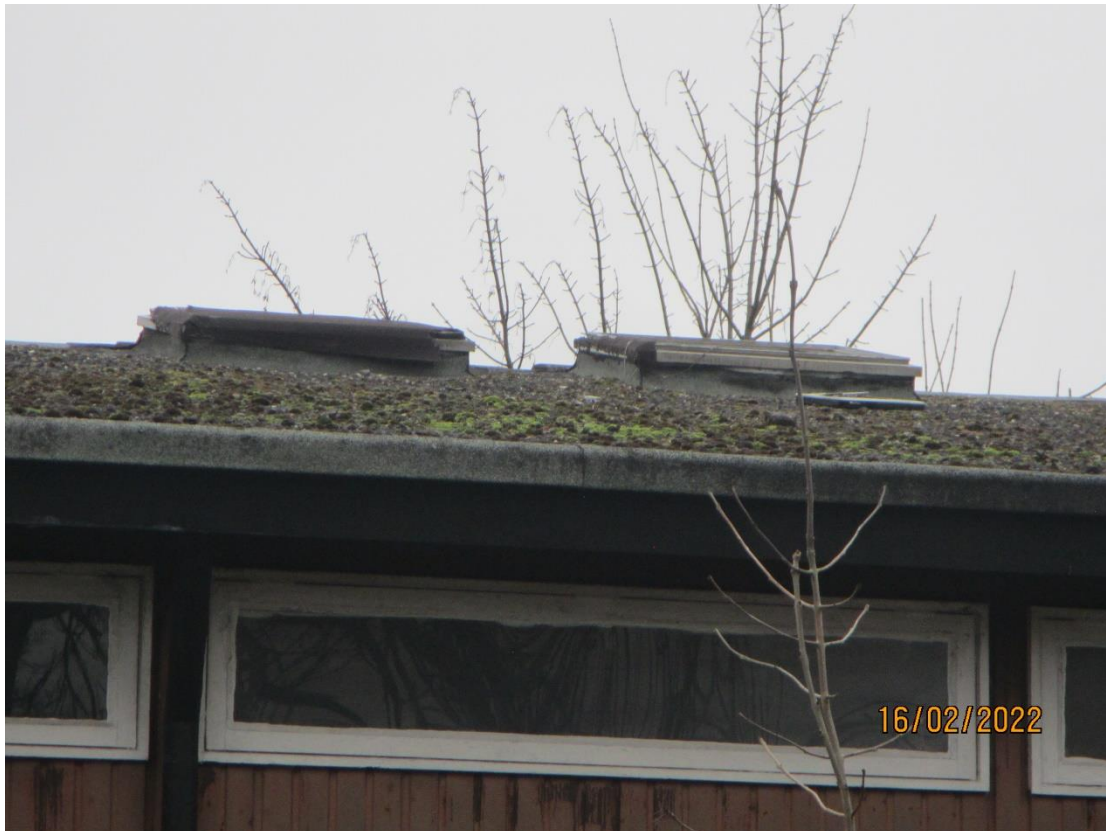
Photograph 3 – Two skylights at the north-western aspect, tightly sealed to the roof with bitumen roof felt, and raised timber roof plank. Wood fascia and windows are also visible.
