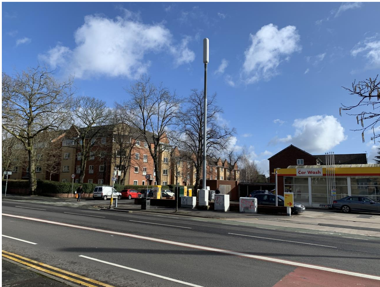
Photograph 1 Existing Mast and associated Equipment (Wilmslow Road)
