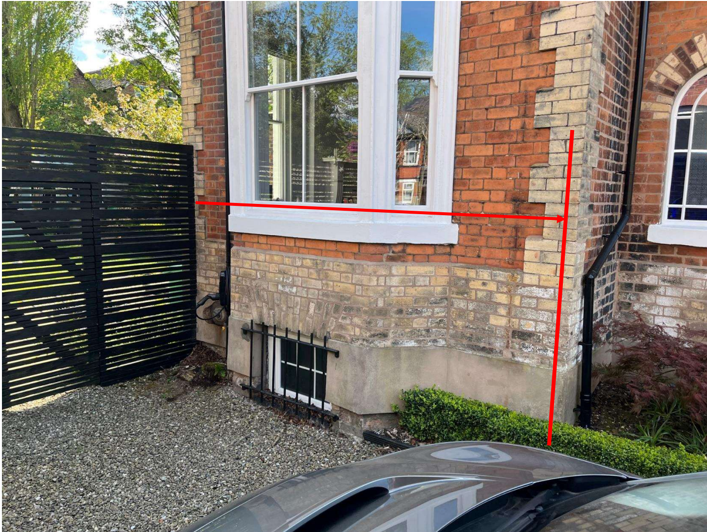
Fence being taken down and re-constructed on this line.
