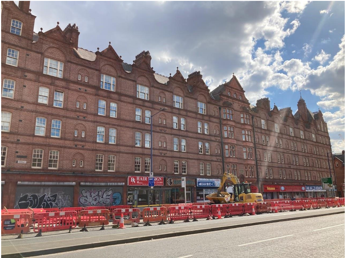
FIGURE 15 – OLDHAM ROAD EXTERNAL ELEVATION
