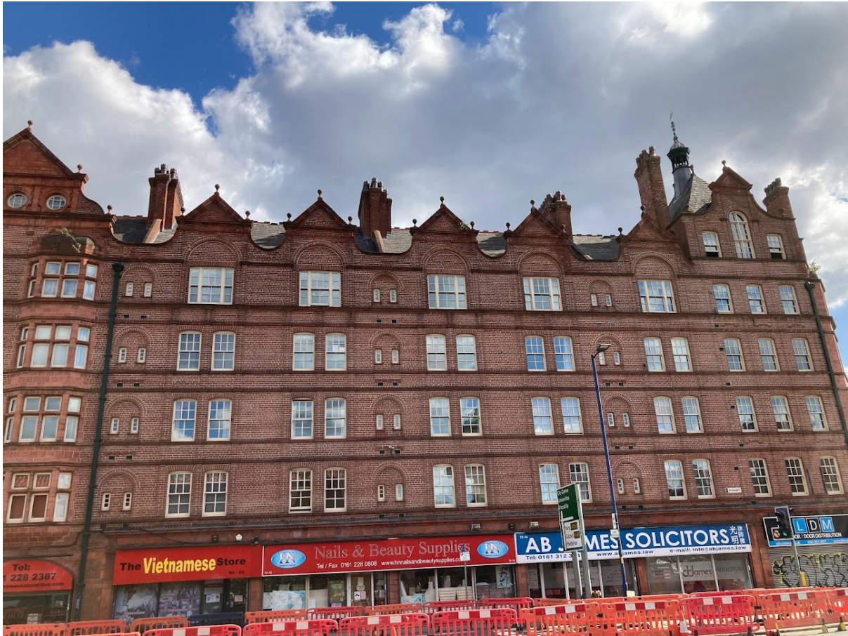
FIGURE 14 – OLDHAM ROAD EXTERNAL ELEVATION
