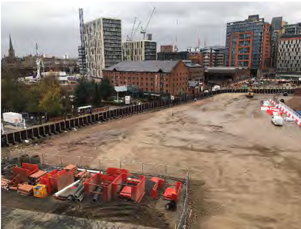
Photograph 2. Extents of piling mat
