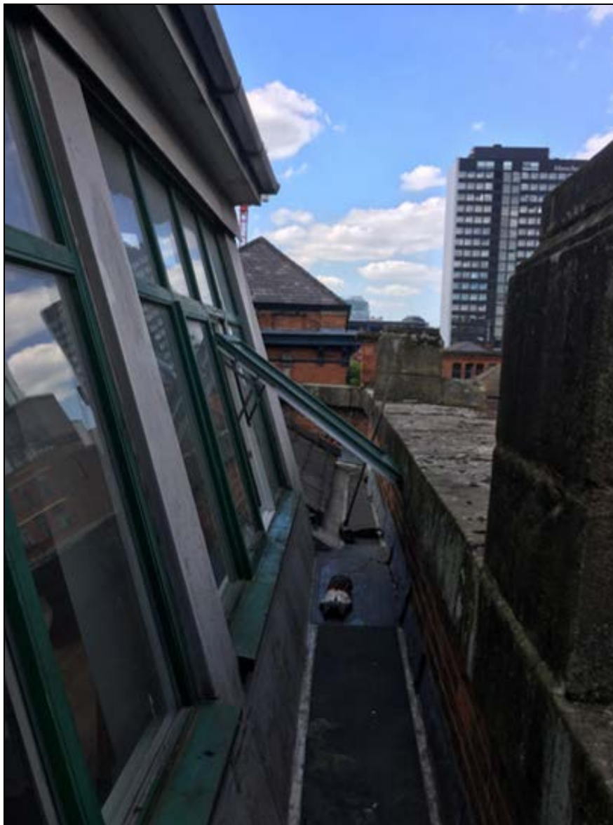
3. The sloping windows of the dormer, set behind the original parapet
