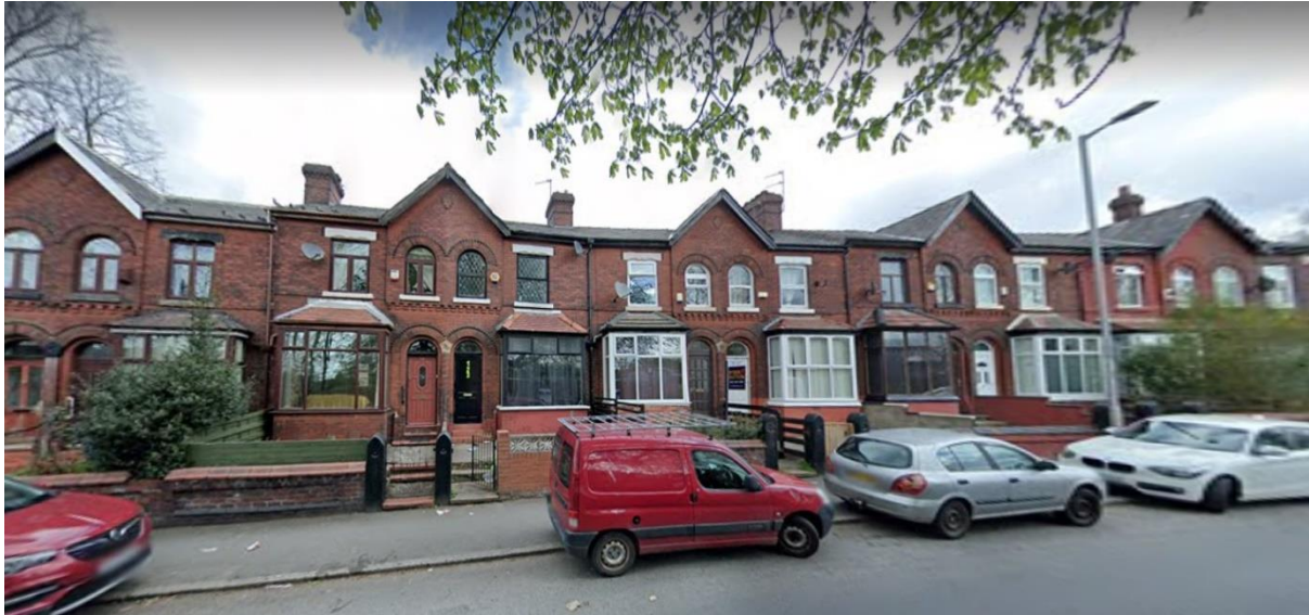
Fig.24: church lane houses directly opposite the site, Google Street View (2022)
