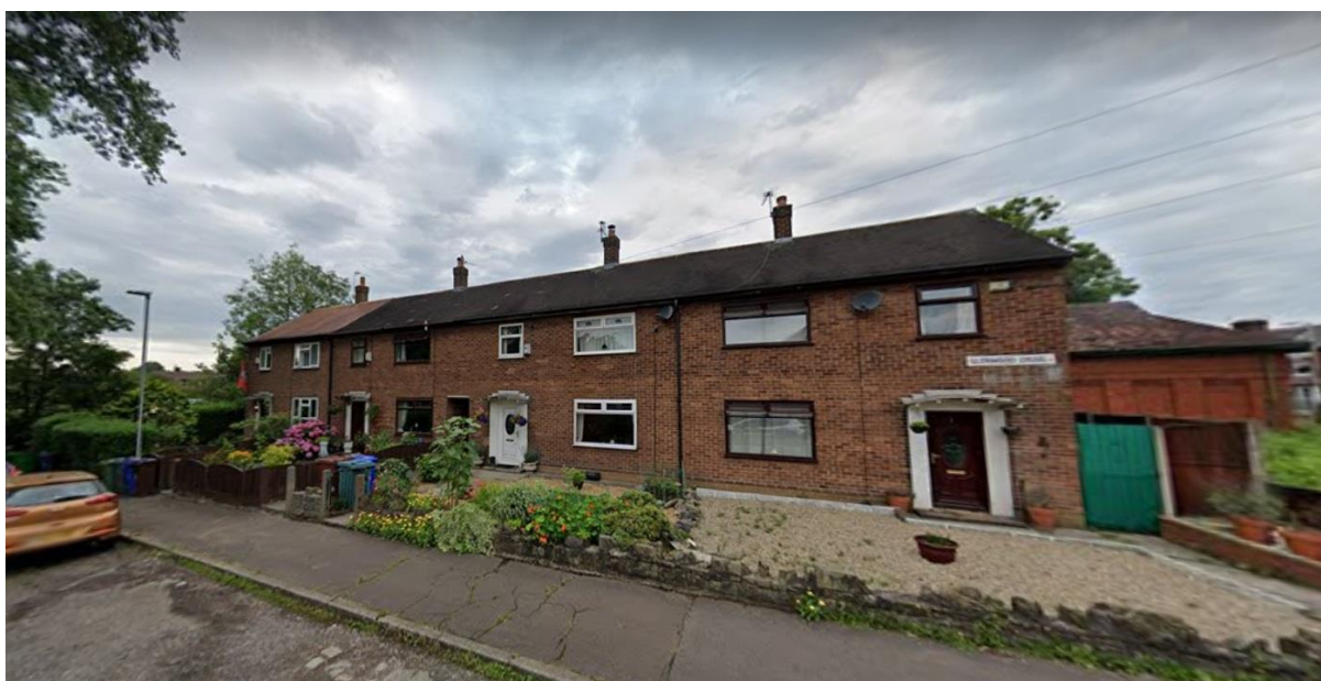
Fig.10: Glenwood Drive double storey houses in east of the site, Google Street View (2022).
