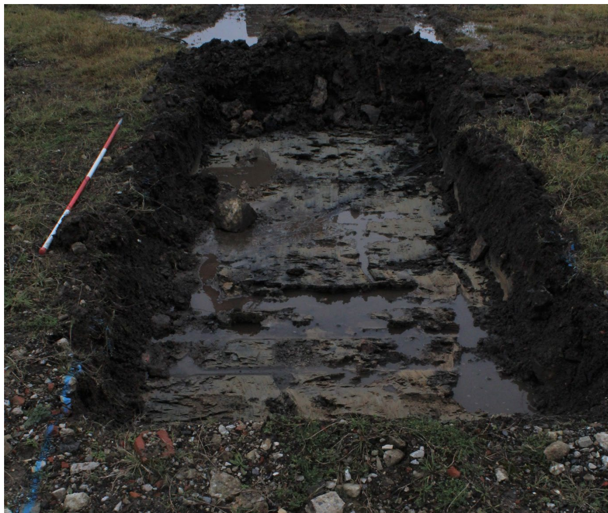
Plate 5: Trench 4, cast-iron pipe
