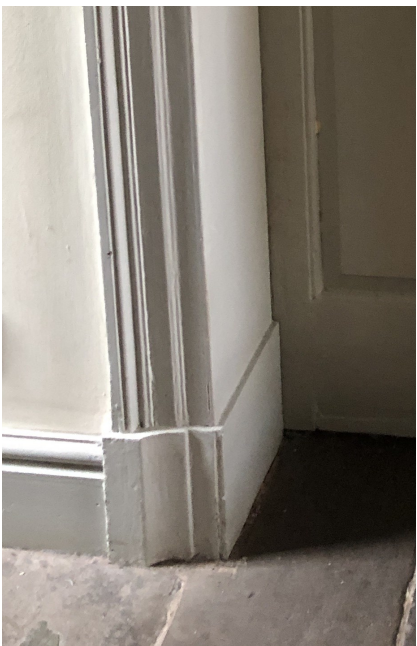
8. Existing architrave detailing in Moor Cottage
