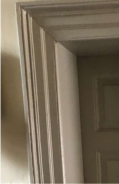
8. Existing architrave detailing in Moor Cottage
