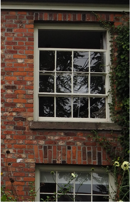
11. Existing glazing to be upgraded in existing frames
