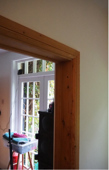
5. Existing opening between Kitchen and Hallway (non original)
