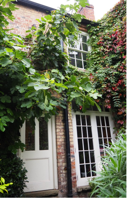
12. Existing non-original external doors to be removed
