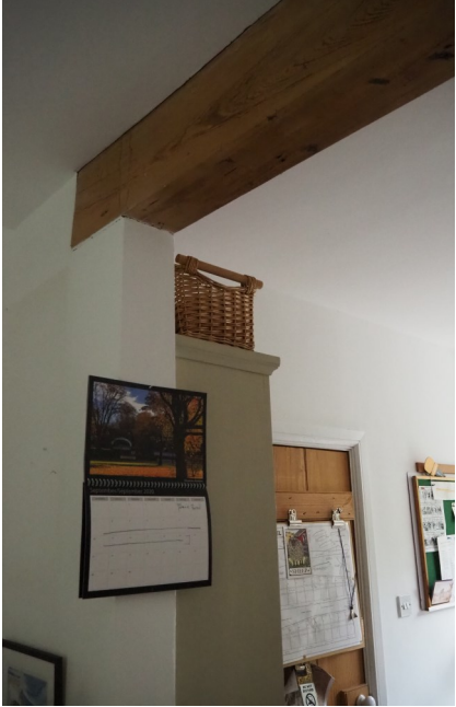
3. Existing opening between Kitchen and Office
