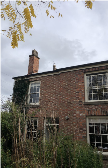
9. Areas of existing fascias/ gutters to be repaired like for like
