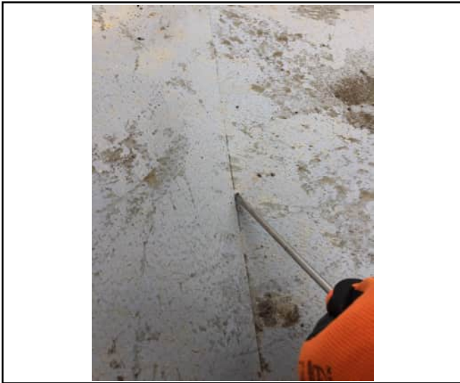
Pick and probe test carried out
