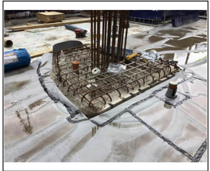
Overview of seal to pile cap
