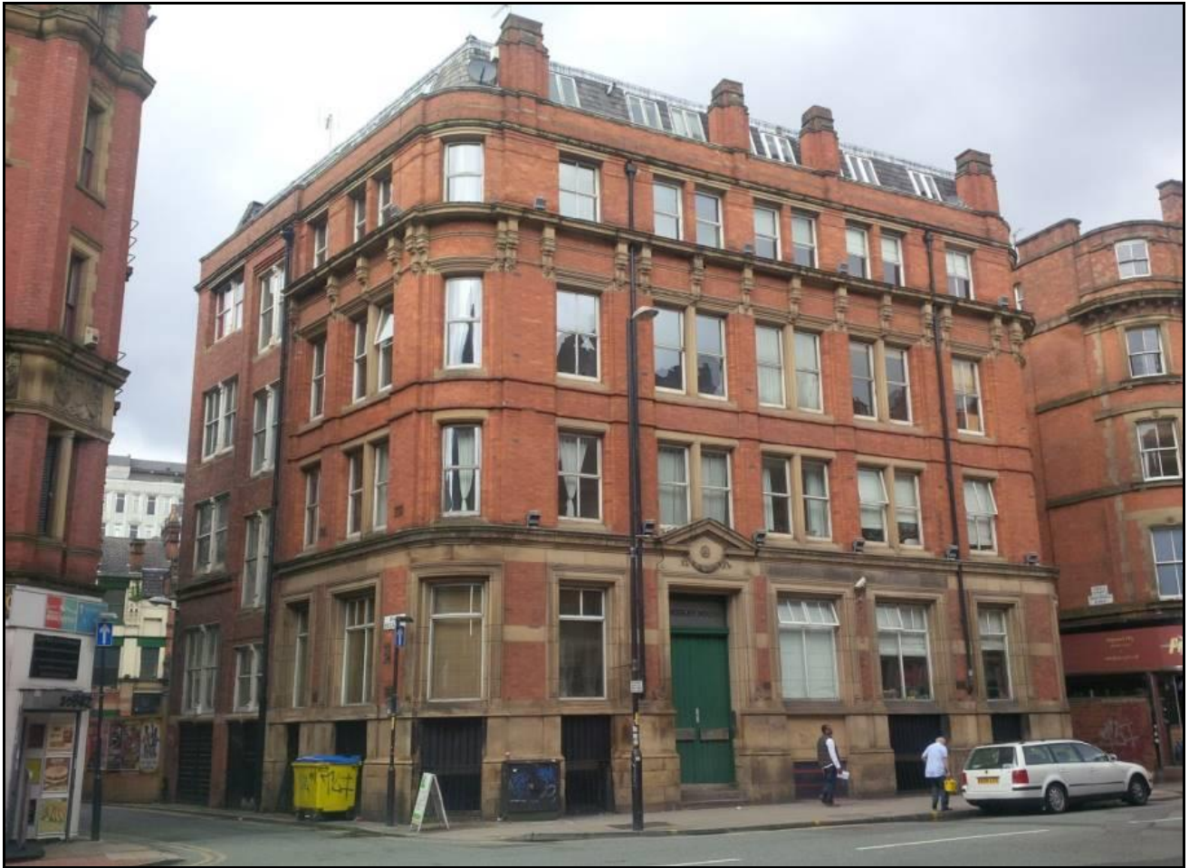
Figure 5) Kingsley House facade (13/15 Newton Street)
