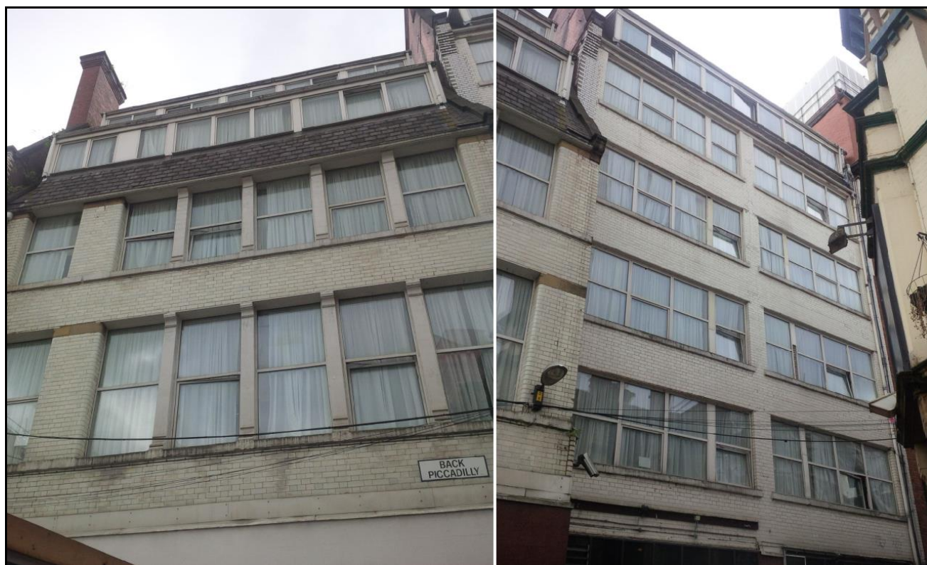
Figure 7) Back Piccadilly facades of nos 55/57 and nos 51/53
