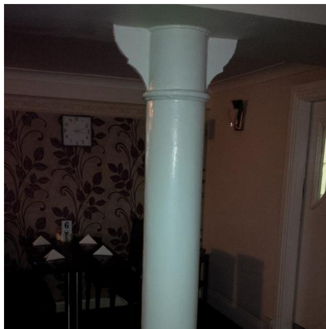
Figure 9) Cast iron column
