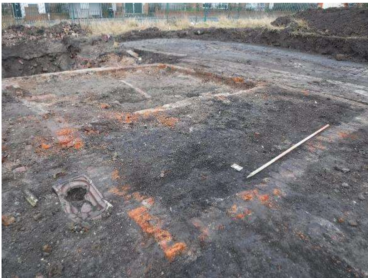
Figure 32: A south-east facing photograph showing the above-ground extension. Scale 1x2m in 0.5m graduations.
