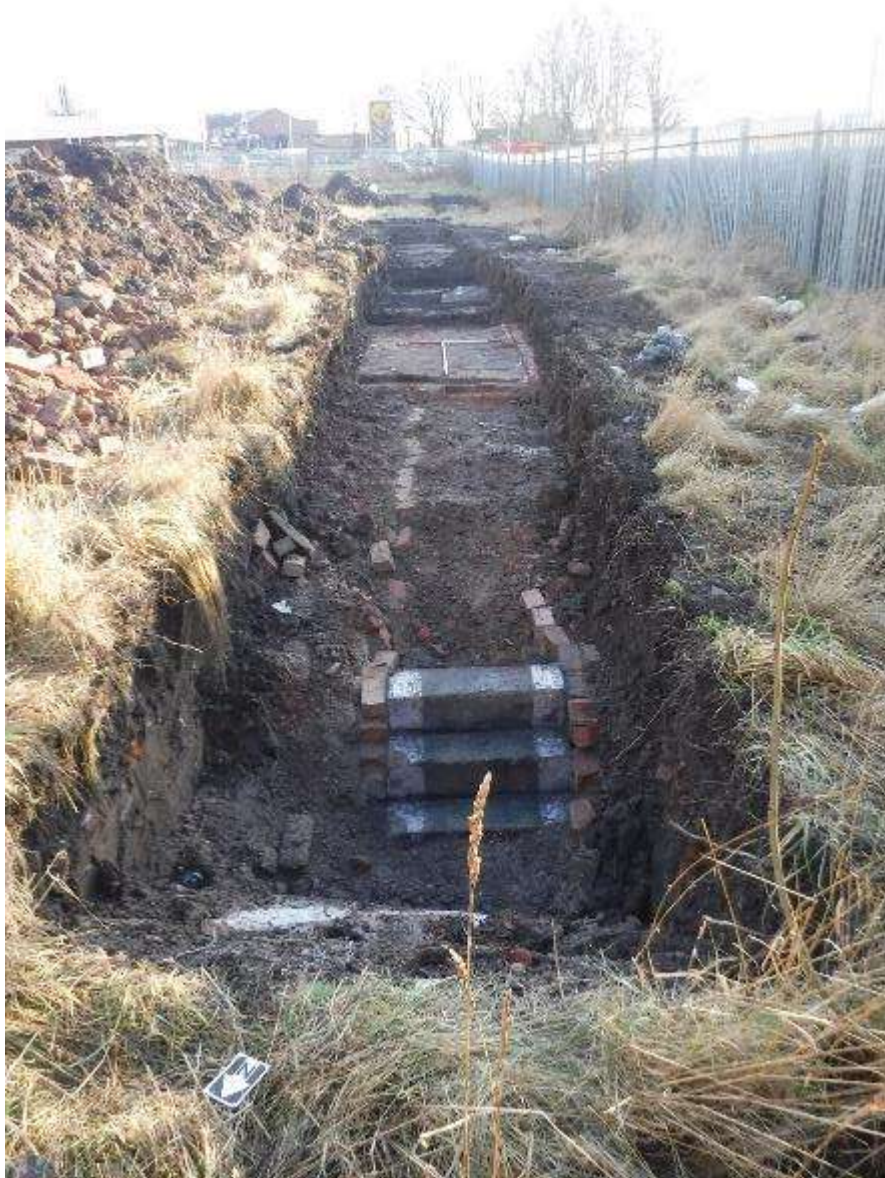
Figure 3: A south-east facing photograph showing Trench 1 with steps {122} in the foreground. Scale 2x 1m in 0.5m graduations.
