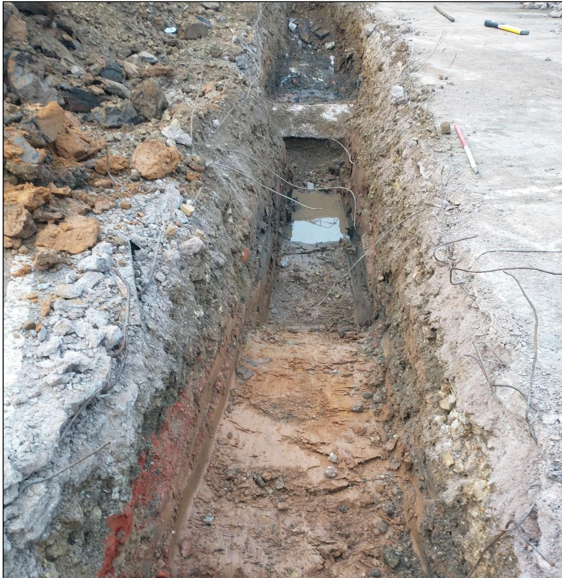
Plate 22: Trench 3 looking east
