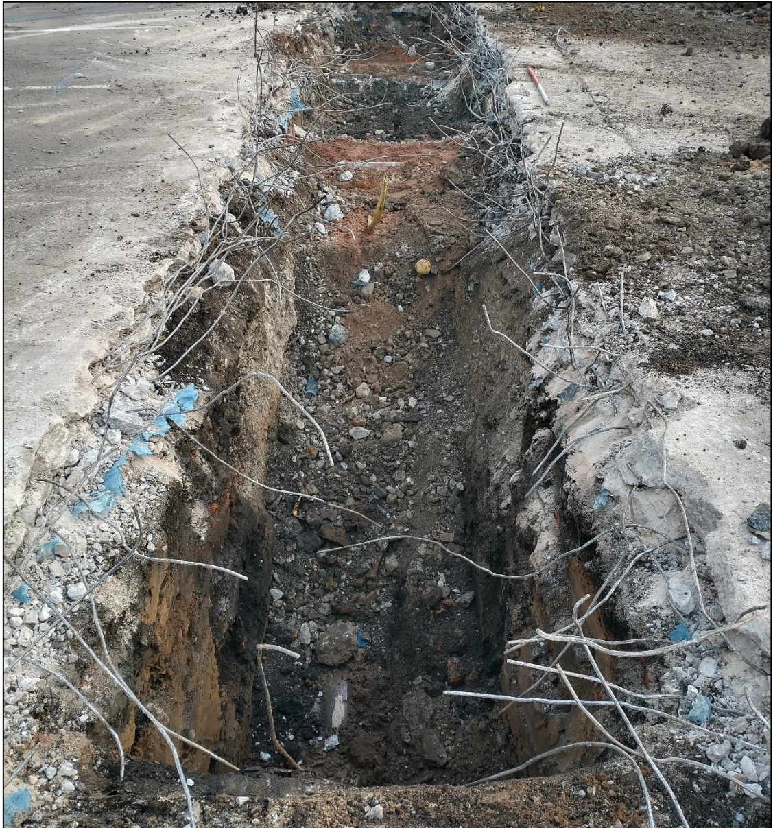
Plate 26: Trench 6 looking northeast
