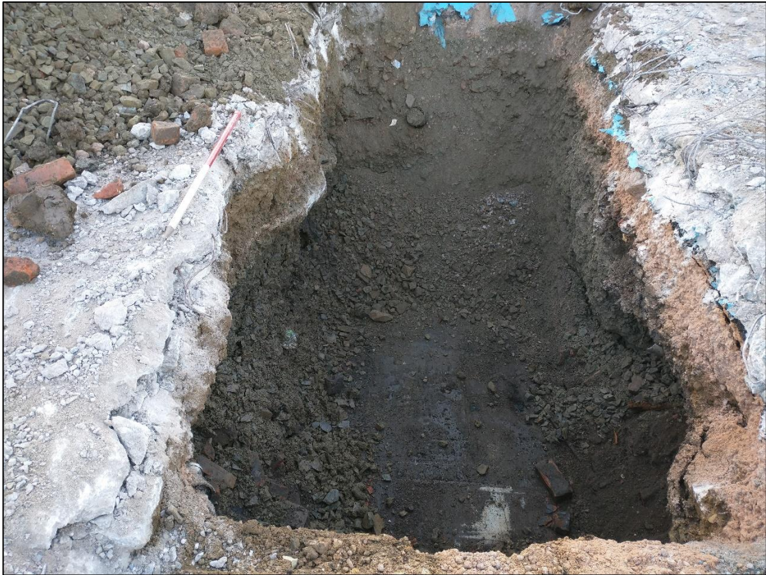
Plate 21: Trench 2 looking southwest
