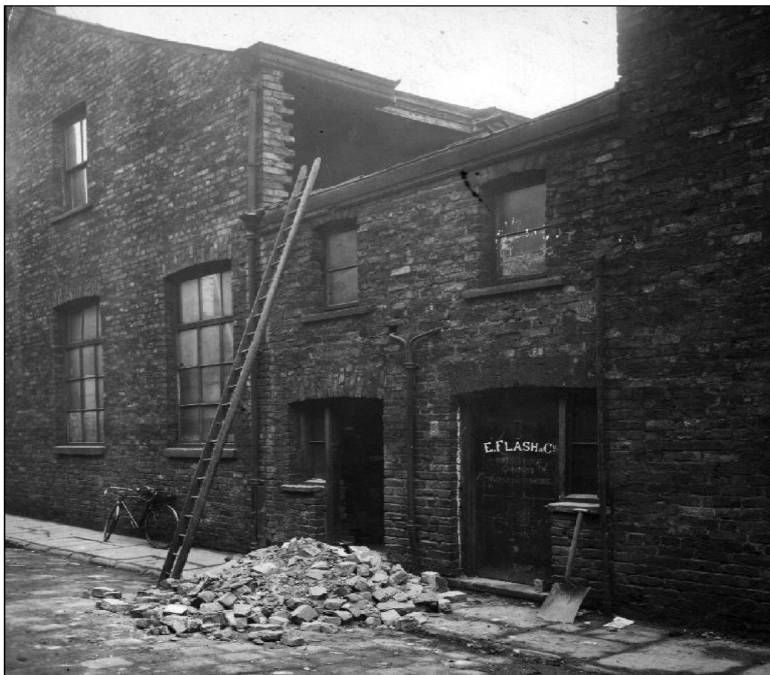
Plate 13: Photograph taken of Nightingale Street in 1920, courtesy of Manchester Local Image Collection
