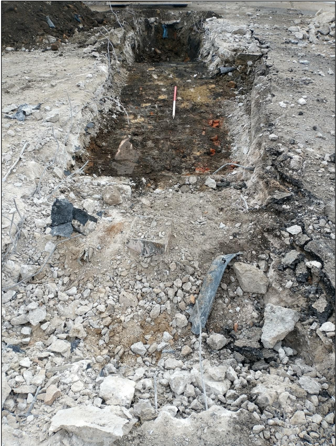
Plate 20: Trench 1 looking southeast, stanchion in foreground
