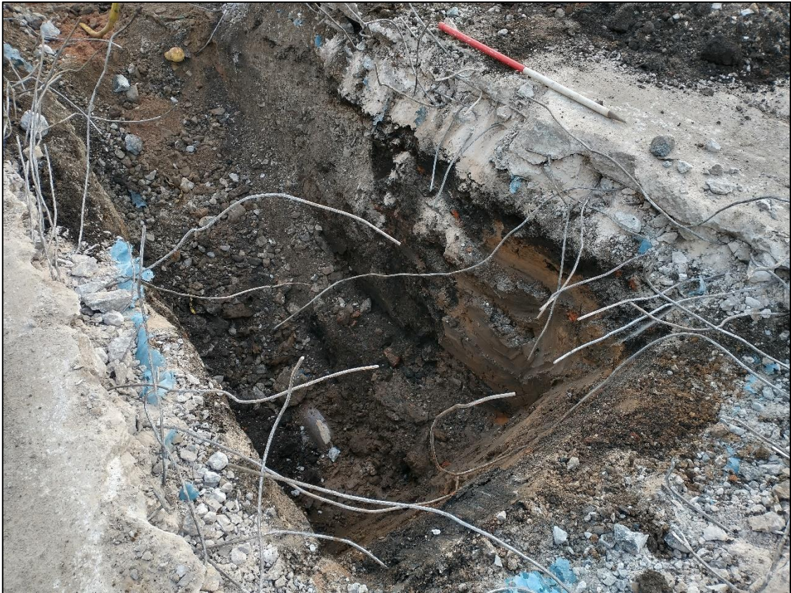
Plate 27: Sewer pipe at the southwest end of trench 6
