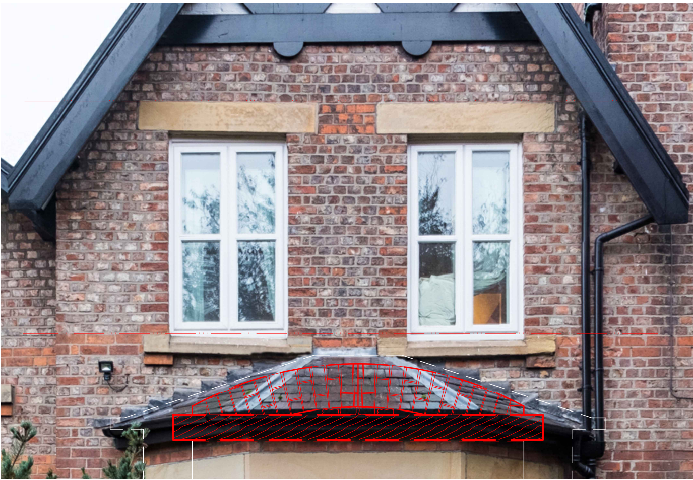
Existing Part West Elevation Photograph with Arch Overlay Not to Scale
