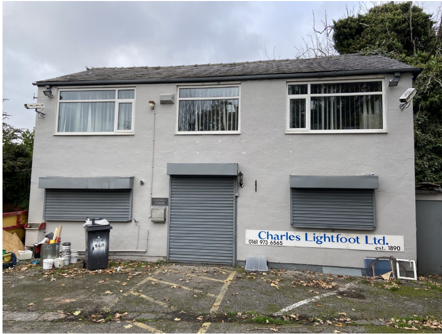
Existing building to be demolished
