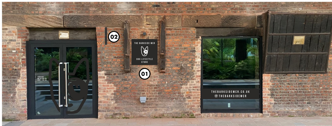
Blade Sign in situ (alongside additional signage for reference)
