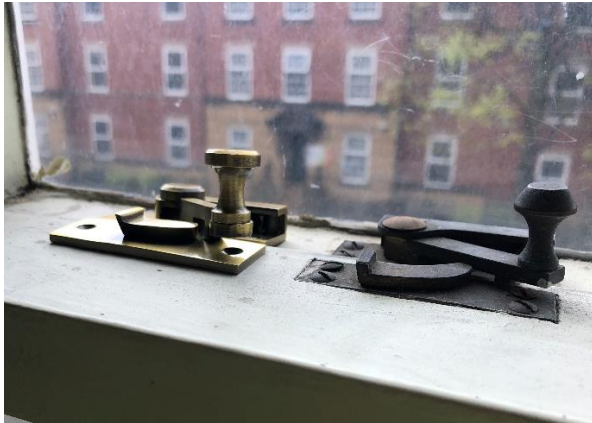
Figures 4 & 5. (above) Photographs of the proposed replacement window ironmongery (sash fasteners and sash lifts) in the finish 'Antique Brass'
