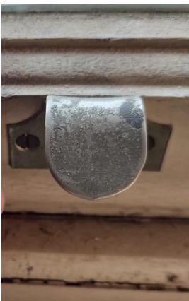
Figures 1 & 2. (above) Photographs of the current window sash fasteners, several of which are no longer functional.
