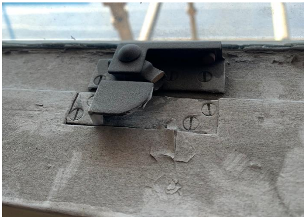
Figures 1 & 2. (above) Photographs of the current window sash fasteners, several of which are no longer functional.
