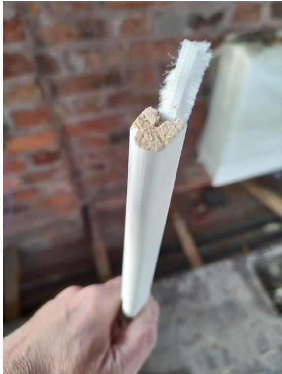
Figures 8 & 9. (above) Photographs showing the proposed timber staff bead with rebated brush draft strips.
