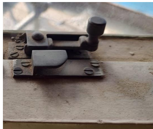
Figures 1 & 2. (above) Photographs of the current window sash fasteners, several of which are no longer functional.
