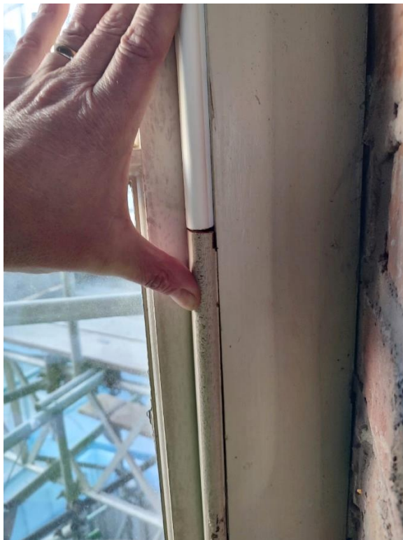
Figures 6 & 7. (above) Photographs of the proposed timber staff beads next to the existing, showing the profile matches like-for-like and the rebated brush draft strip is not visible. Windows and new staff beads will be repainted to match existing.
