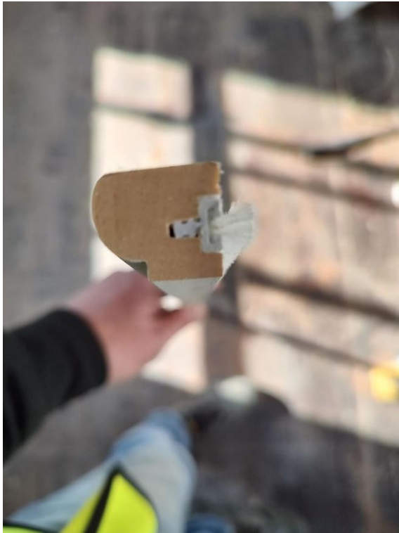
Figures 8 & 9. (above) Photographs showing the proposed timber staff bead with rebated brush draft strips.
