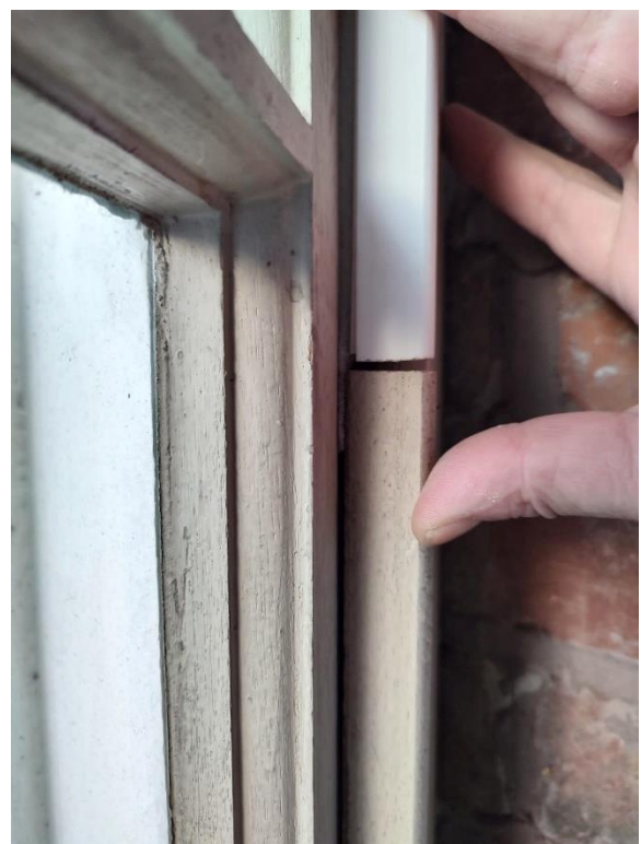
Figures 6 & 7. (above) Photographs of the proposed timber staff beads next to the existing, showing the profile matches like-for-like and the rebated brush draft strip is not visible. Windows and new staff beads will be repainted to match existing.
