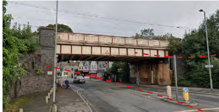
Below; images of Wilmslow Road Railway Bridge; 2019, 1905, 1931
