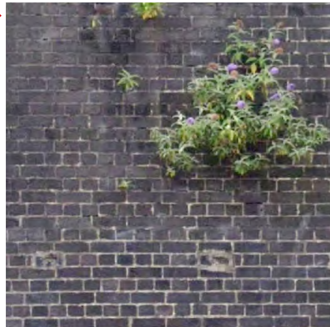
Above; images of Wilmslow Road Railway Bridge
