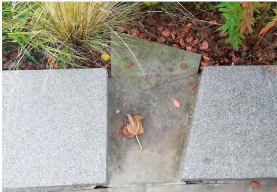
Sustainable Drainage Edge Detail
