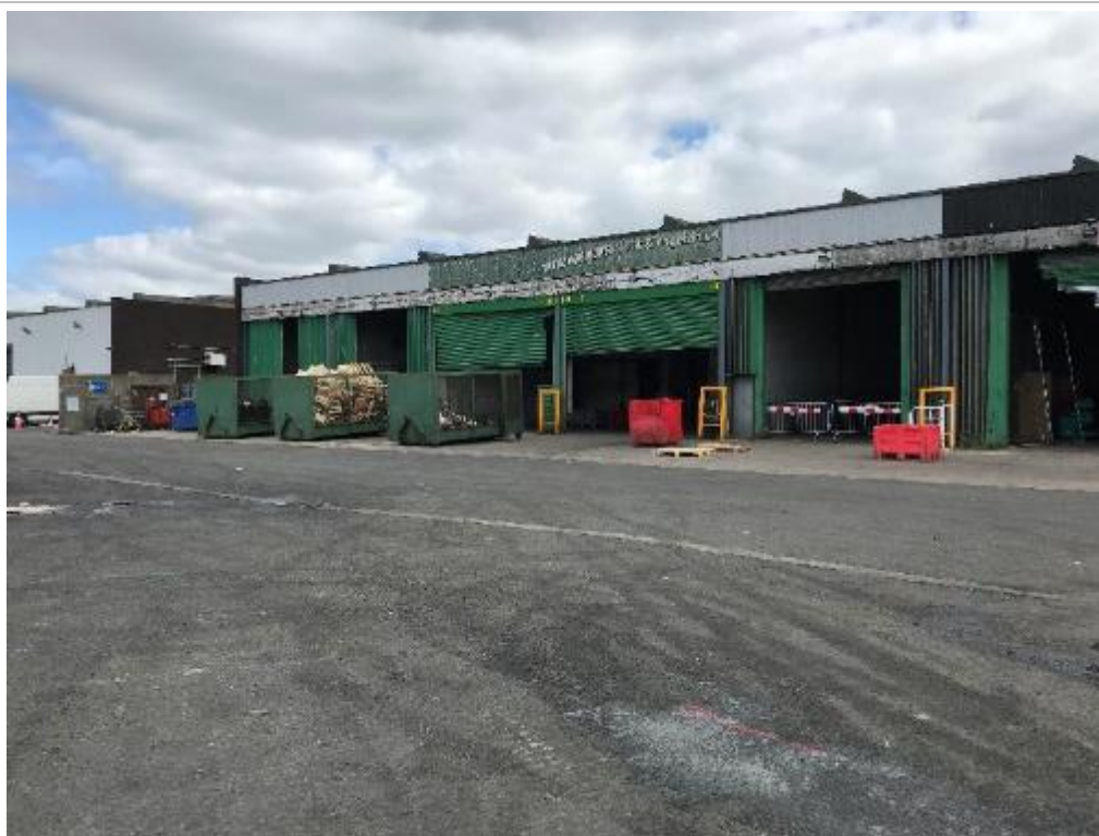
PLATE 2 VIEW OF STORAGE UNITS AT SITE IN BLOCK E
