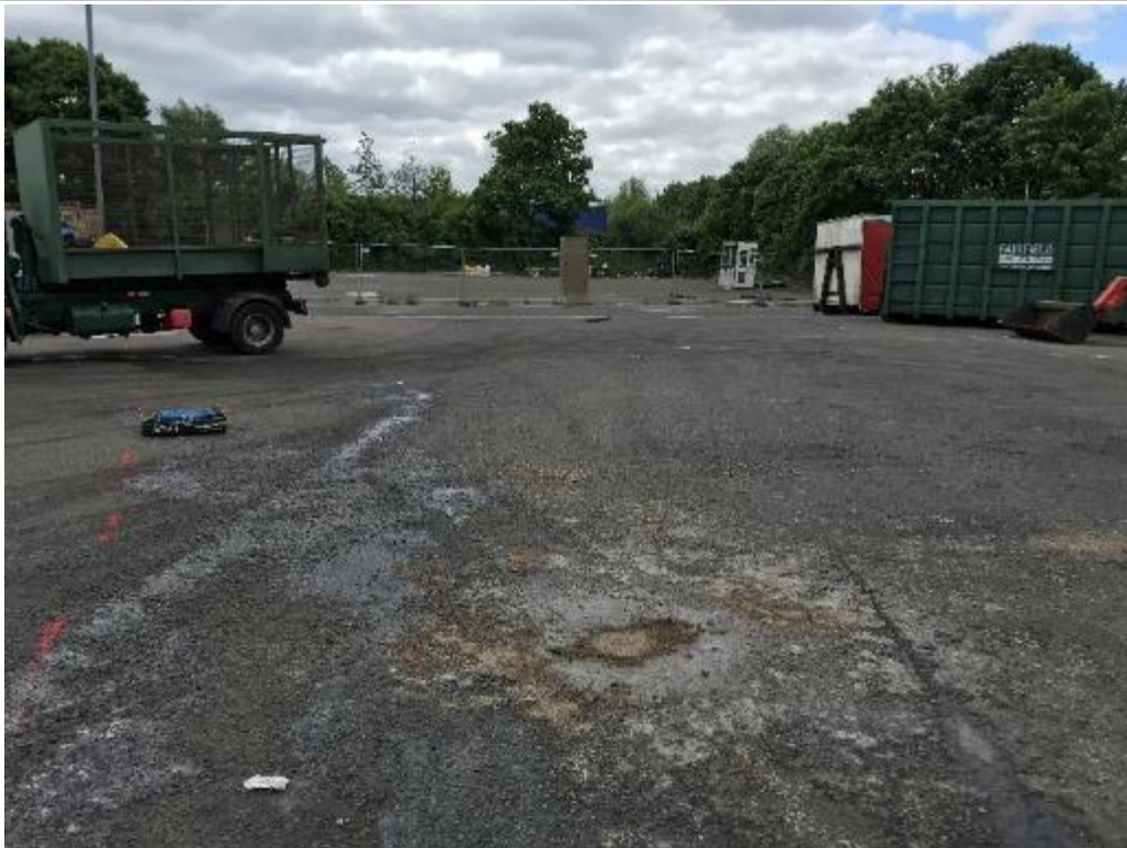
PLATE 4 VIEW OF ASPHALT AREA IN SOUTH EAST OF SITE
