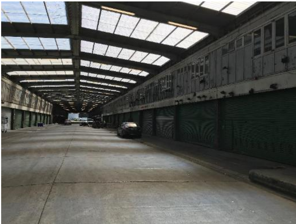
PLATE 3 VIEW OF AREA WITHIN WAREHOUSE D
