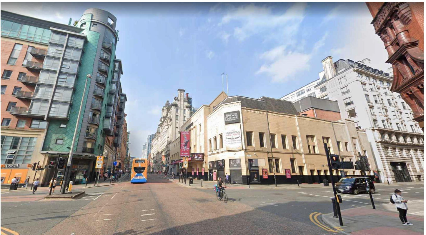
View from corner of Oxford Street and Whitworth Street (Google Street View) – Areas of proposed works obscured by front of theatre building and would not be visible at street level.
