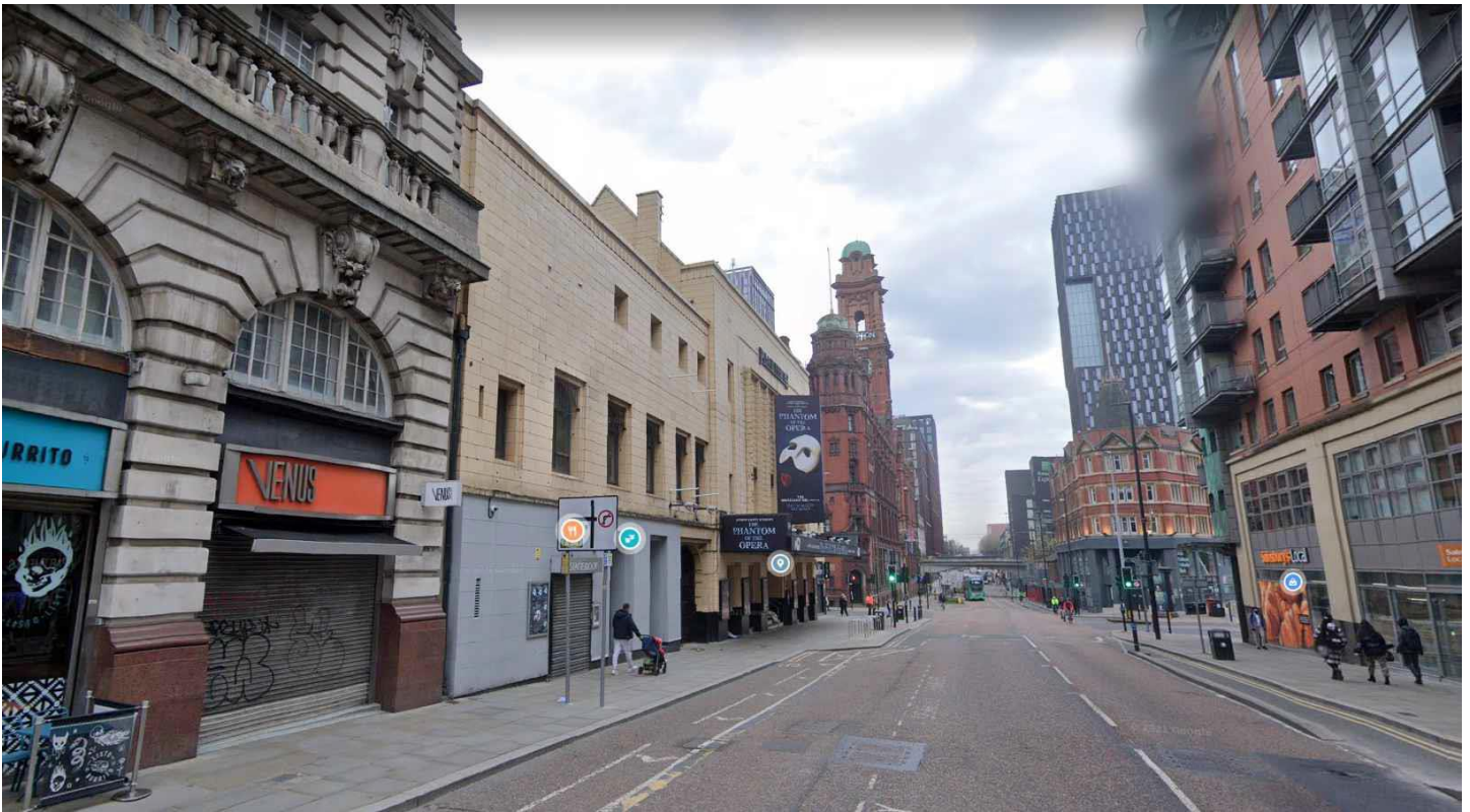
View from Oxford Street (Google Street View) – Areas of proposed works obscured by front of theatre building and would not be visible at street level.
