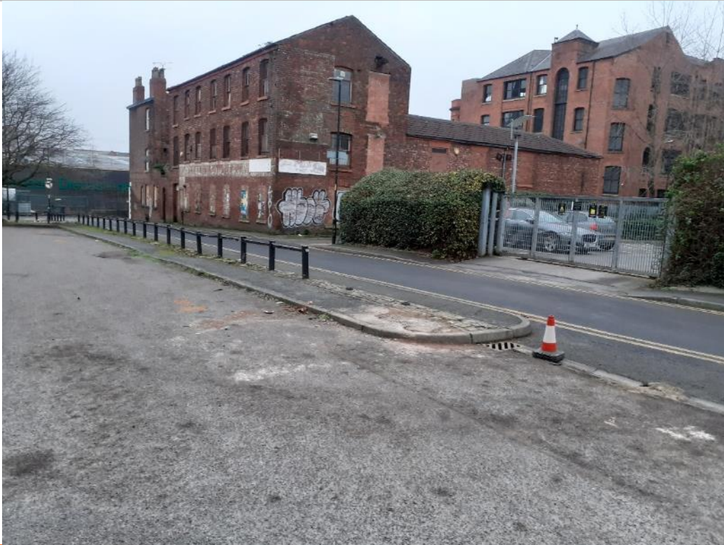
PLATE 1 CAR PARK ENTRANCE – FACING SOUTH WEST
