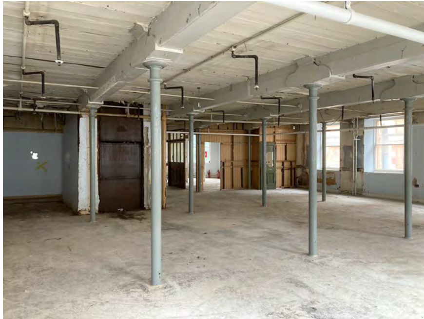
Figure 3: view of the 2nd floor
