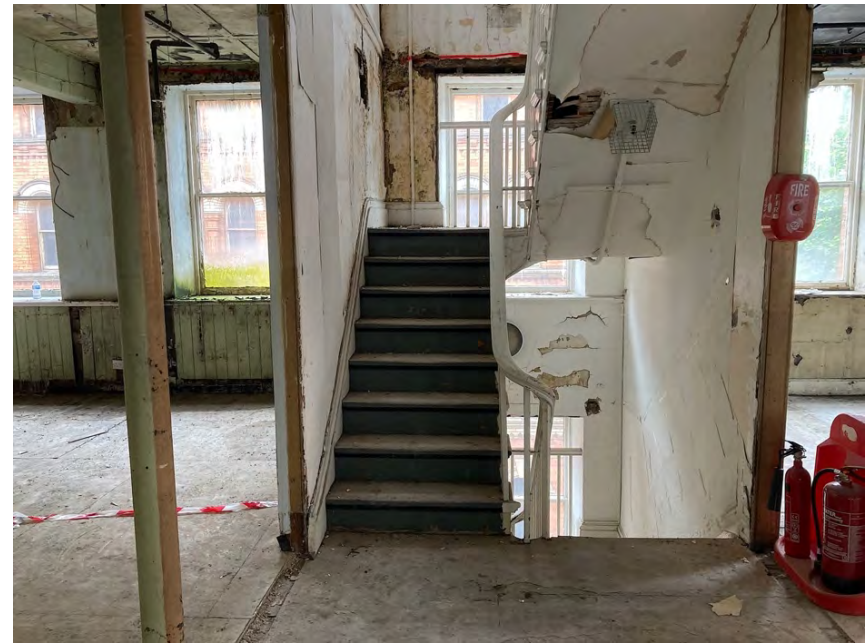
Figure 4: The Stairs &amp; Stairwell
