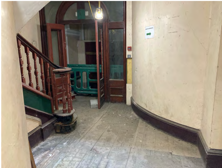
View of the entrance at the foot of the main stair
