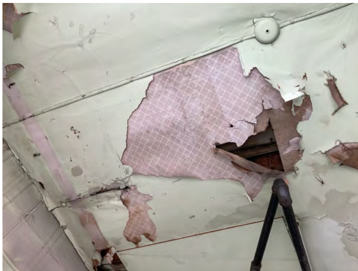
Figure 7: Evidence for patterned ceiling paper (3 rd Floor)
