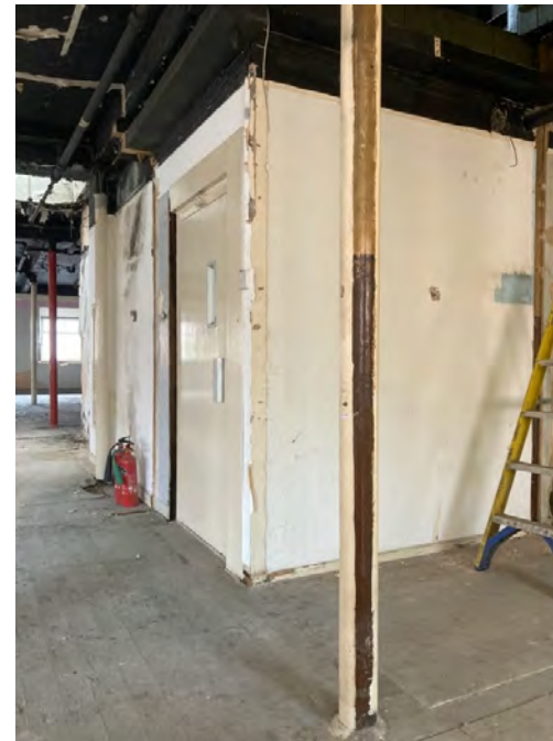
Figure 8: Phase II decoration revealed on iron column on 4 th Floor
