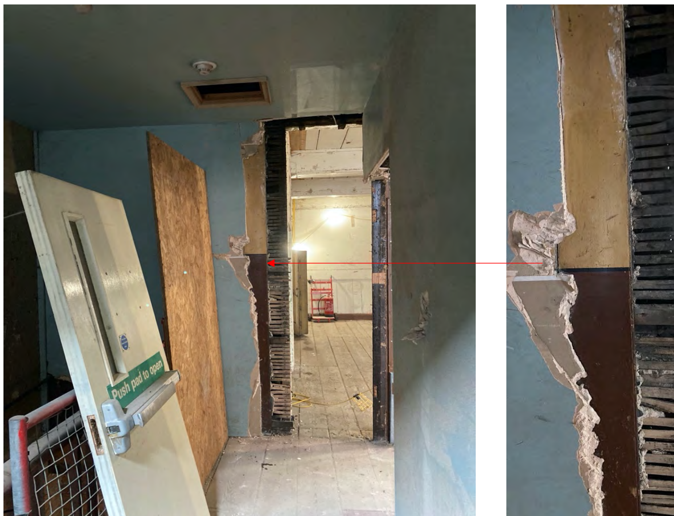
Figure 2: Revealed phase II stud wall on the 1 st Floor
