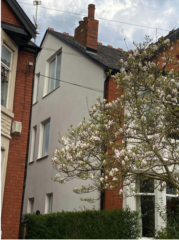
Photographs of 57 Wood Road, Whalley Range, showing external wall insulation system with pale render finish to gable wall, with roof extended over at verge.
