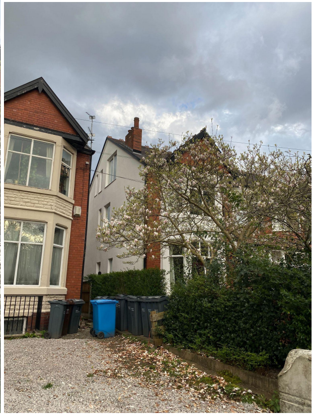
Photographs of 57 Wood Road, Whalley Range, showing external wall insulation system with pale render finish to gable wall, with roof extended over at verge.
