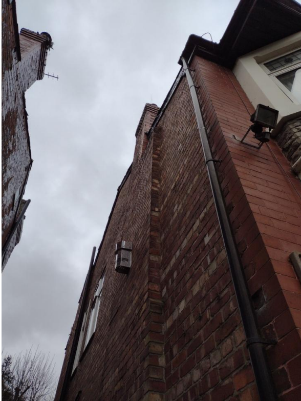
Photograph of gable elevation as viewed from the gated side access leading to the rear garden.
