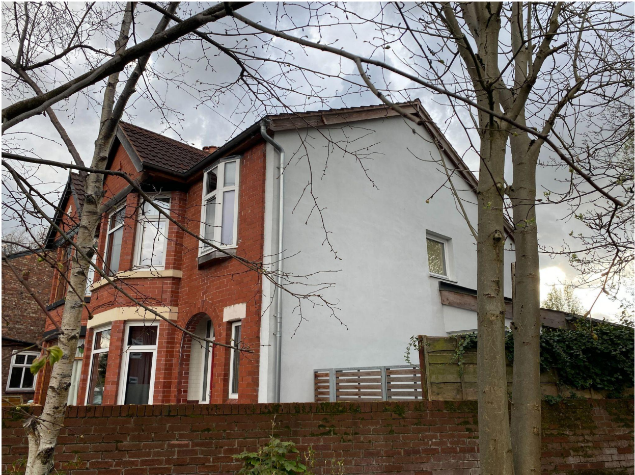
Photograph of 2 Park Drive, Whalley Range, showing external wall insulation system with pale render finish to gable wall, with roof extended over at verge.
