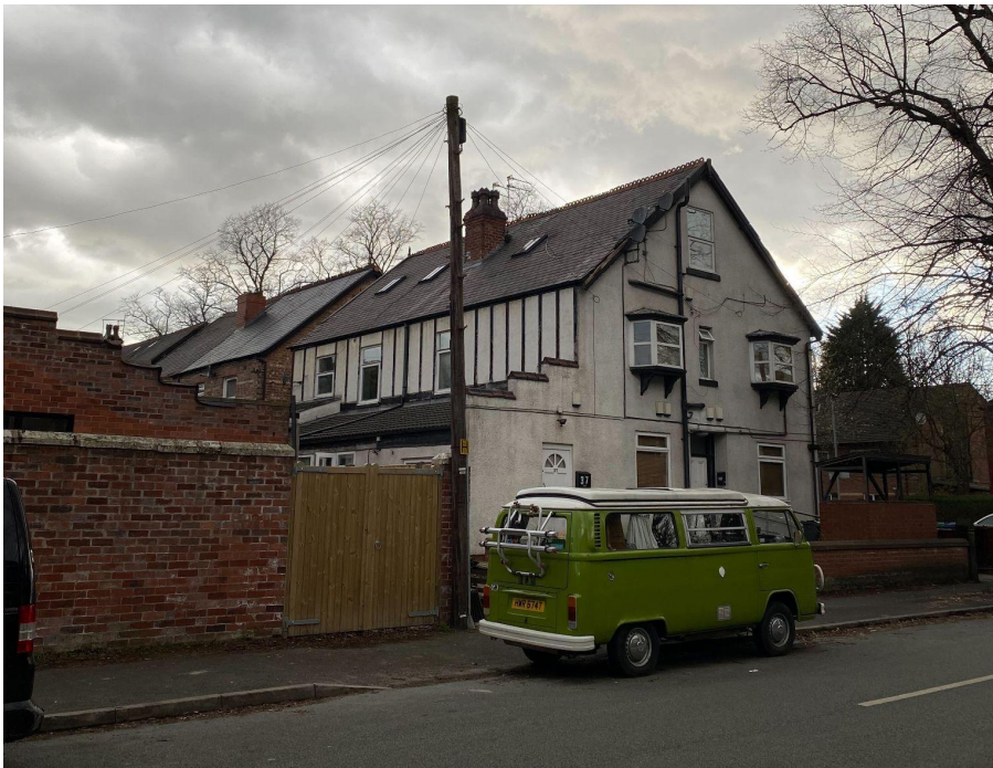
Photograph of 37 Russell Road, Whalley Range, showing a mix of pale render and red brick to front elevation with white render on side and rear elevations.
