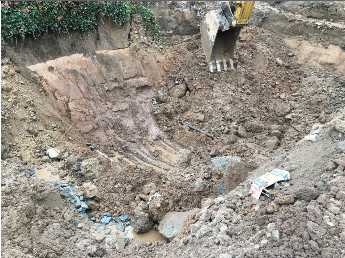
Plate No. 1: Fuel tank excavation
