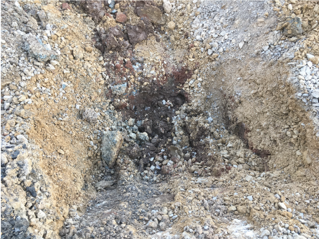
Plate No. 1: VAL05 Excavation
