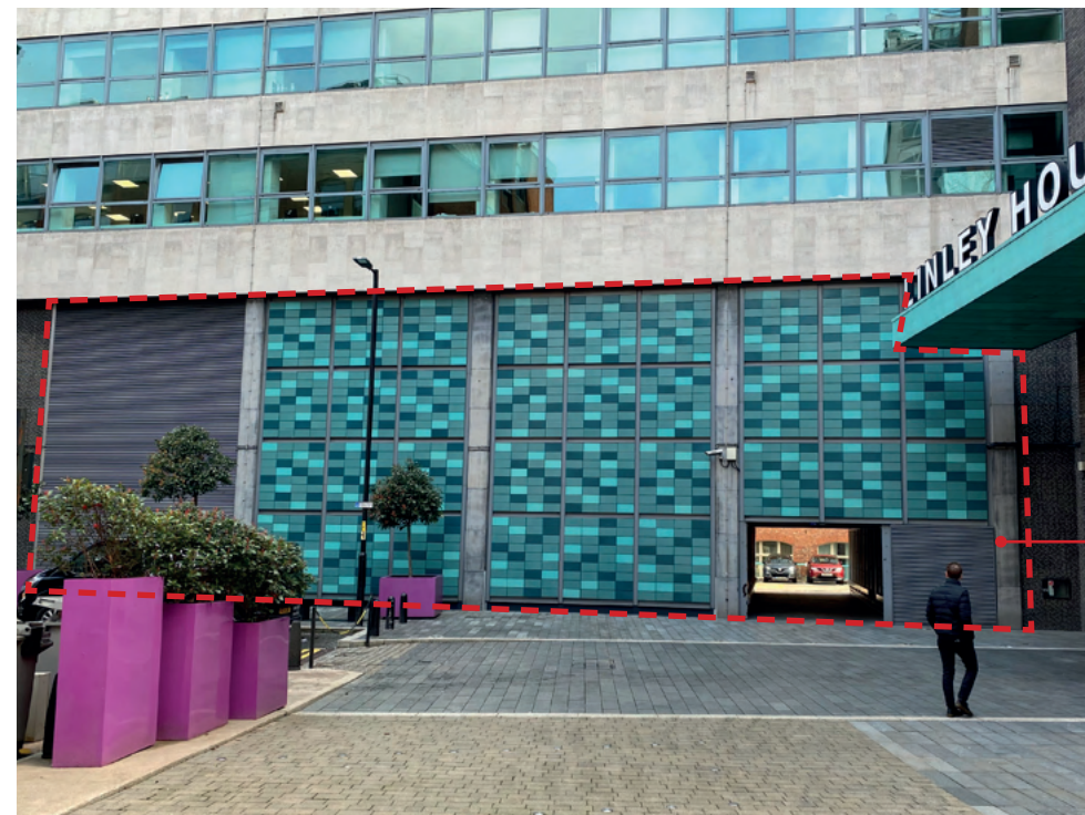
Existing building facade
