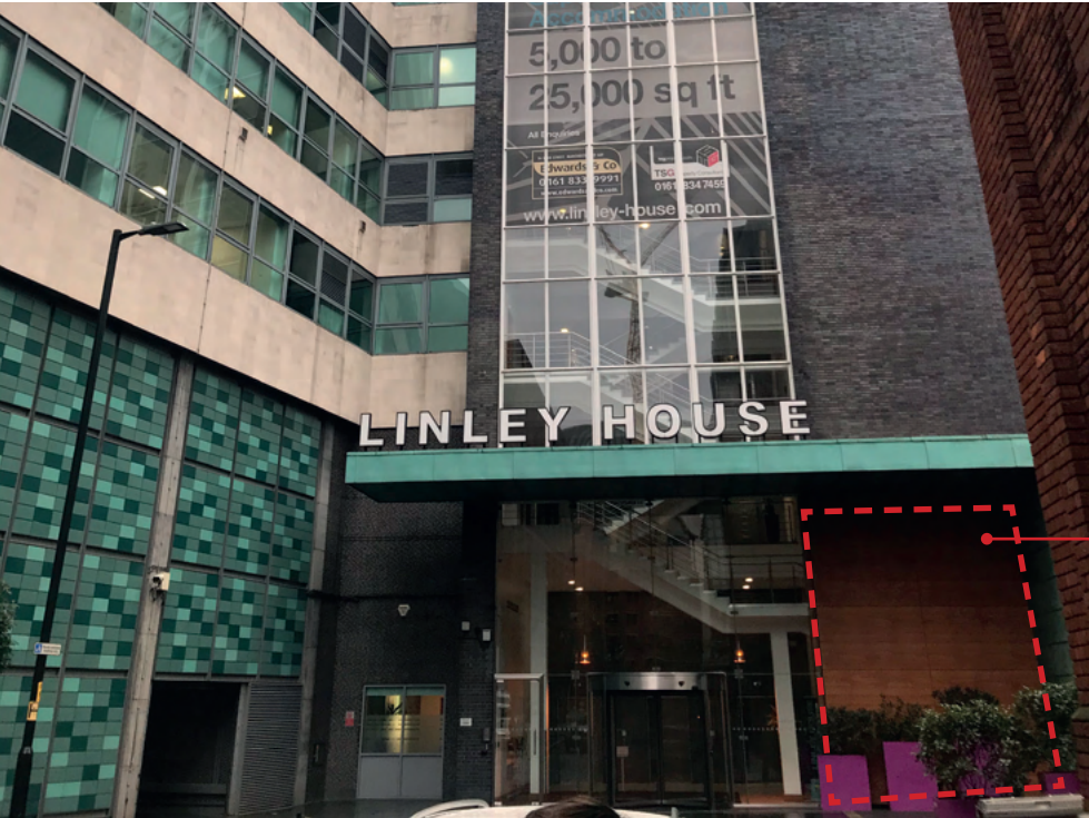
Existing building facade
