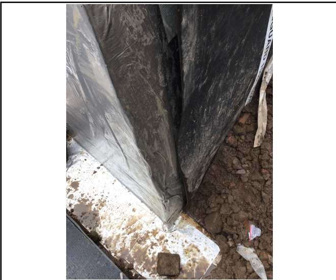
Final corner of D5 complete
