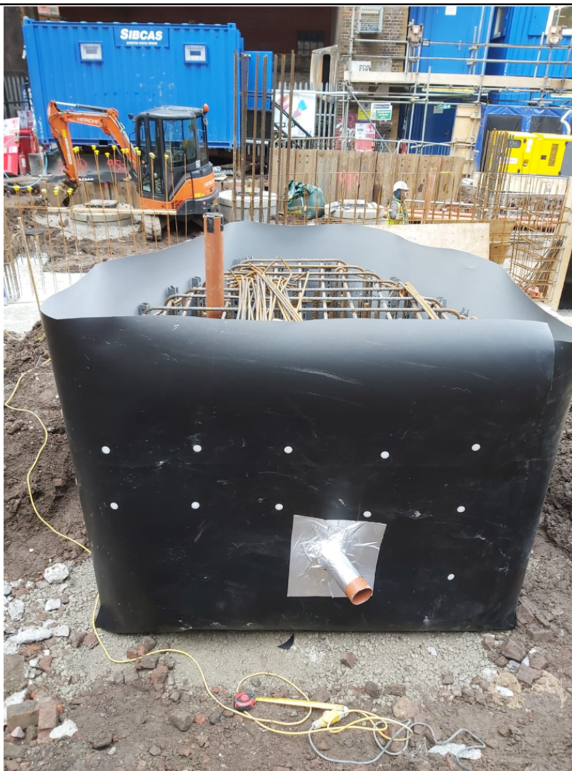
Overview of pile cap sealed
