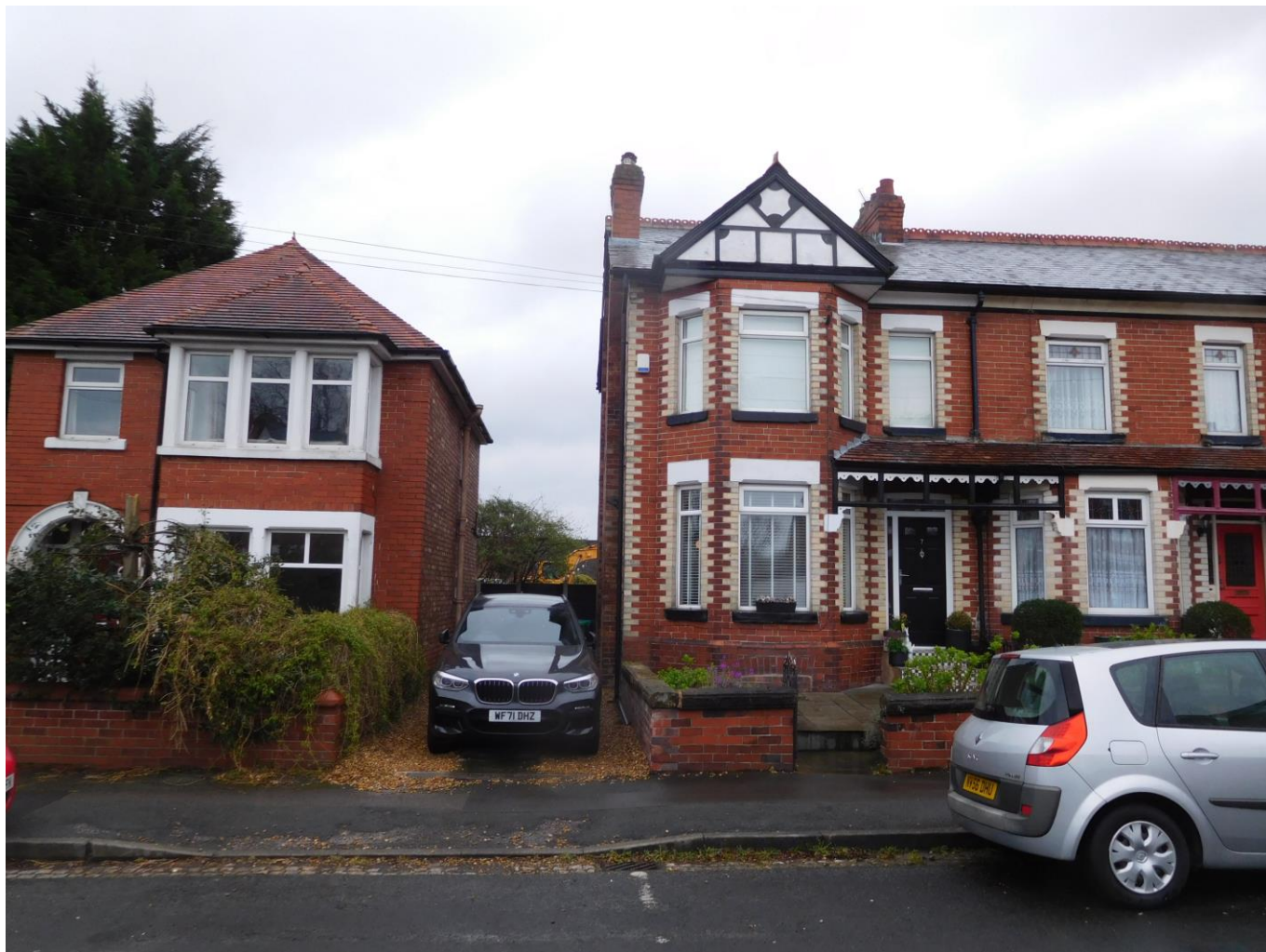
Photograph 1 Application Site as viewed from Chapel Road, Source: Officer's site photographs 05.04.2022
