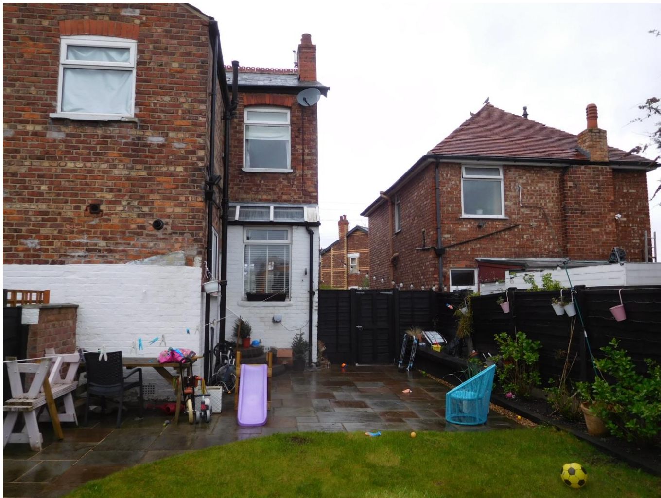
Photograph 2 Rear of both 7 Chapel Road (left hand side) and 7a Chapel Road (right hand side).
